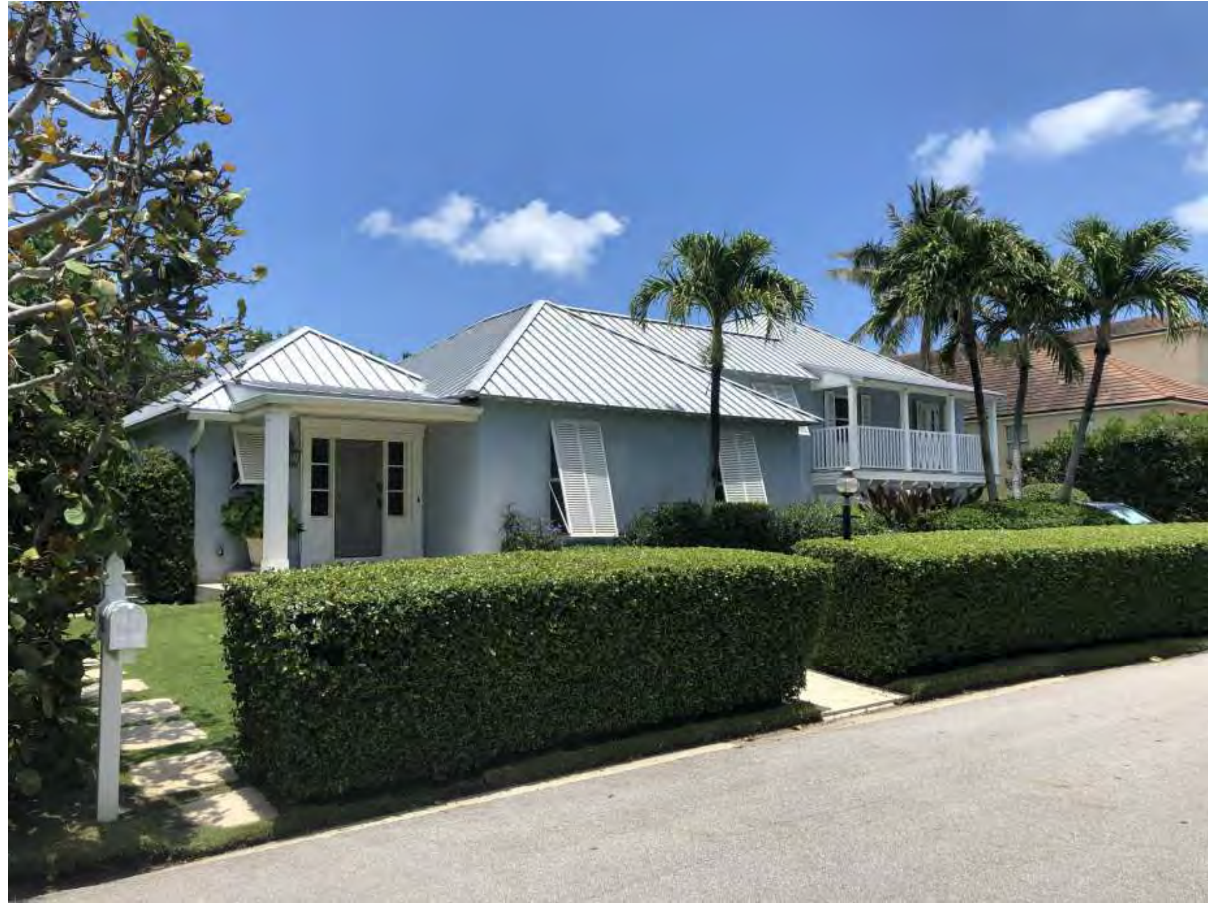
A EXISTING FRONT YARD - VIEW FROM REEF ROAD L-3
