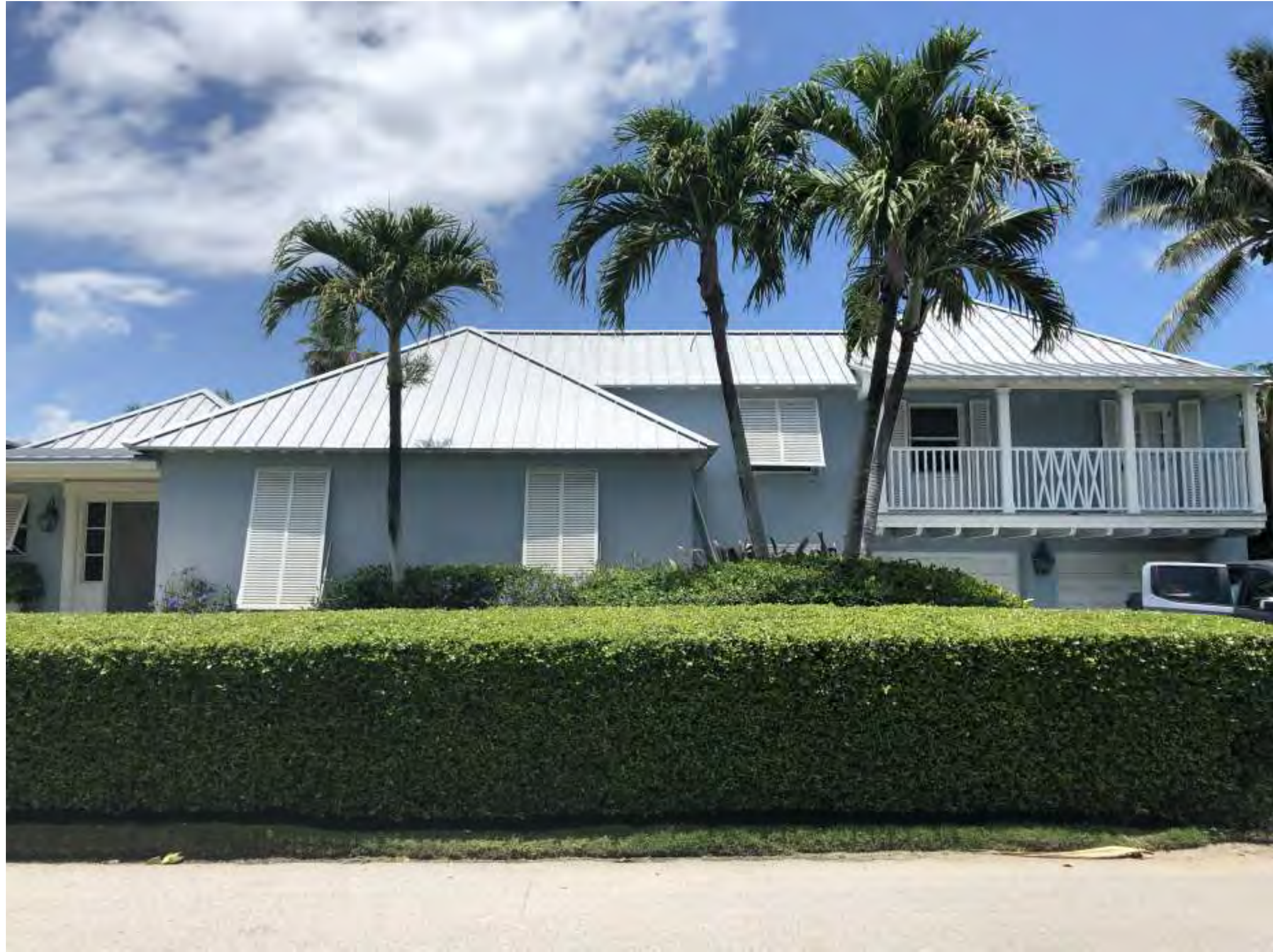
B EXISTING FRONT YARD - VIEW FROM REEF ROAD L-3
