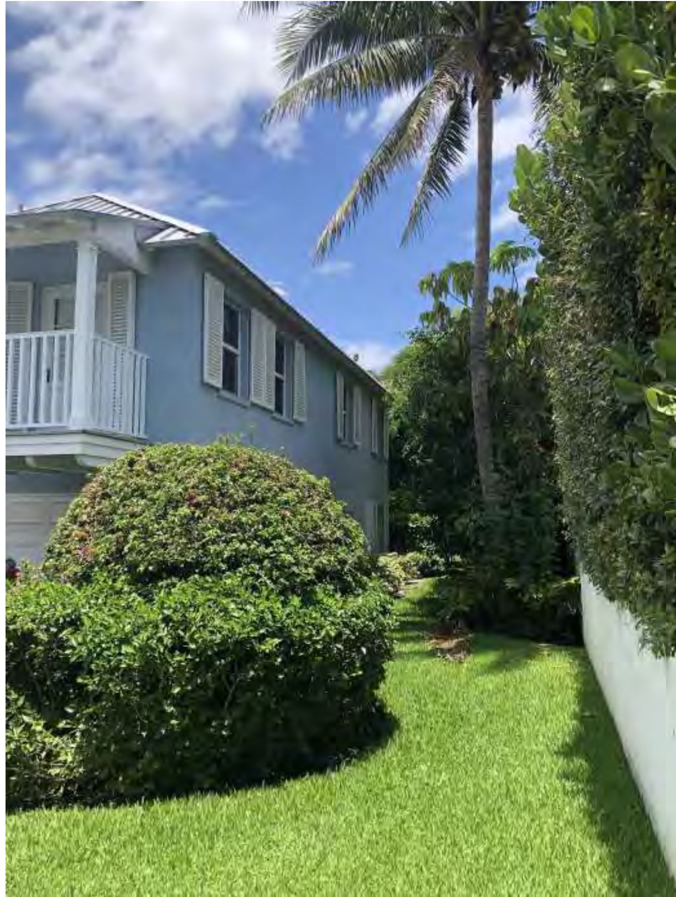
E L-4 EXISTING SIDE YARD EAST
