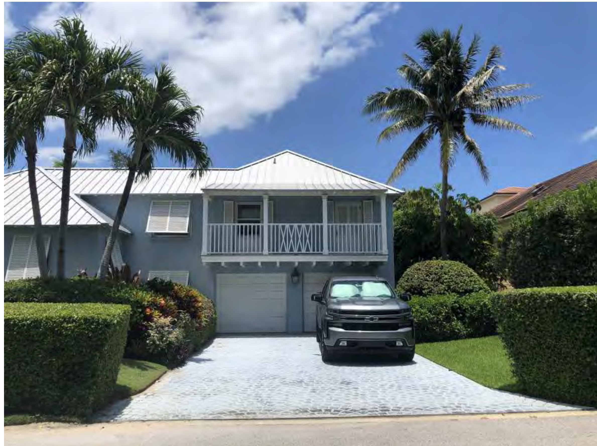
C EXISTING DRIVEWAY - VIEW FROM REEF ROAD L-3
