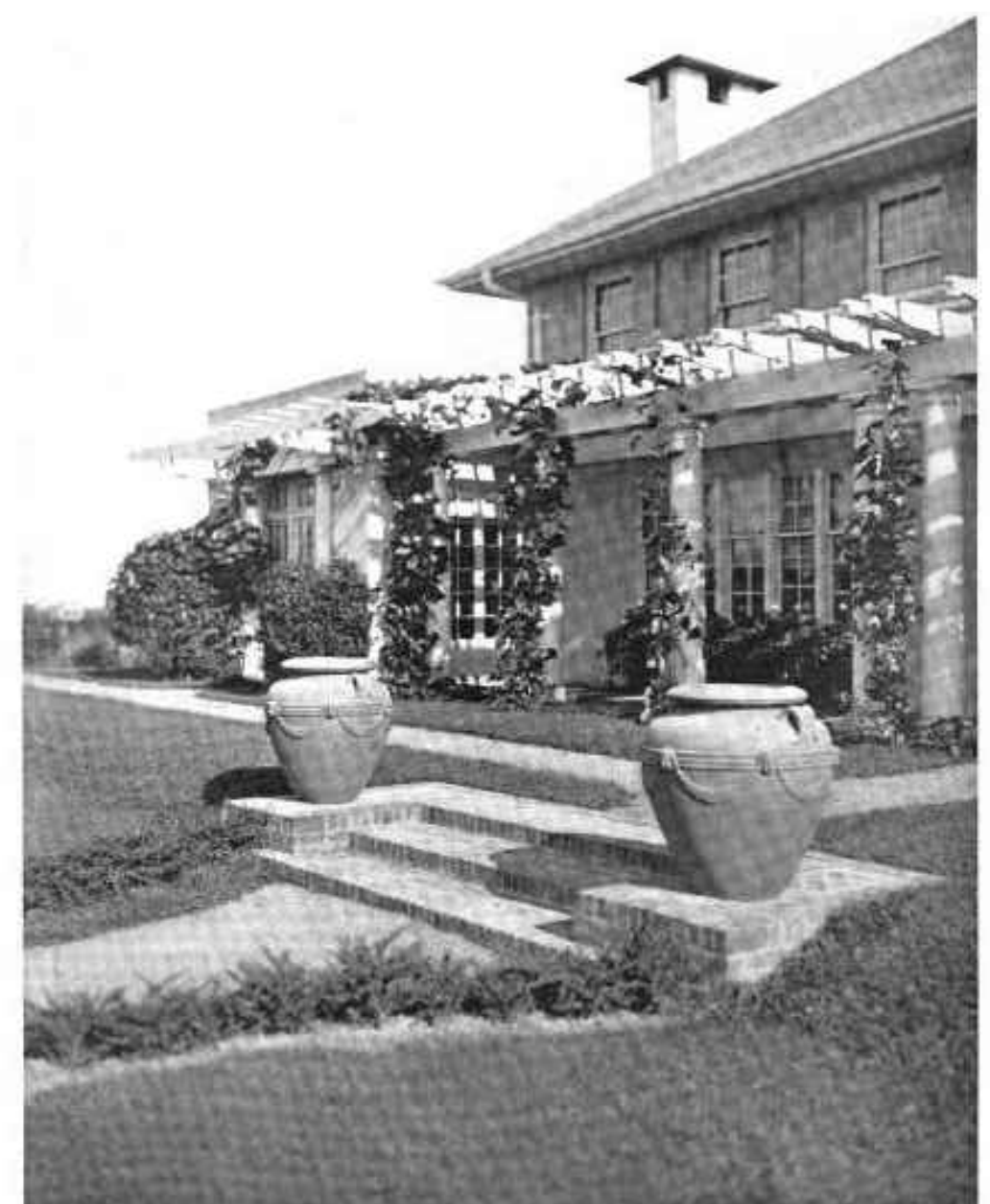
RESIDENCE OF DR. FREDK K. HOLLISTER, EAST HAMPTON, L.I. ALBRO & LINDBERG, Architects
