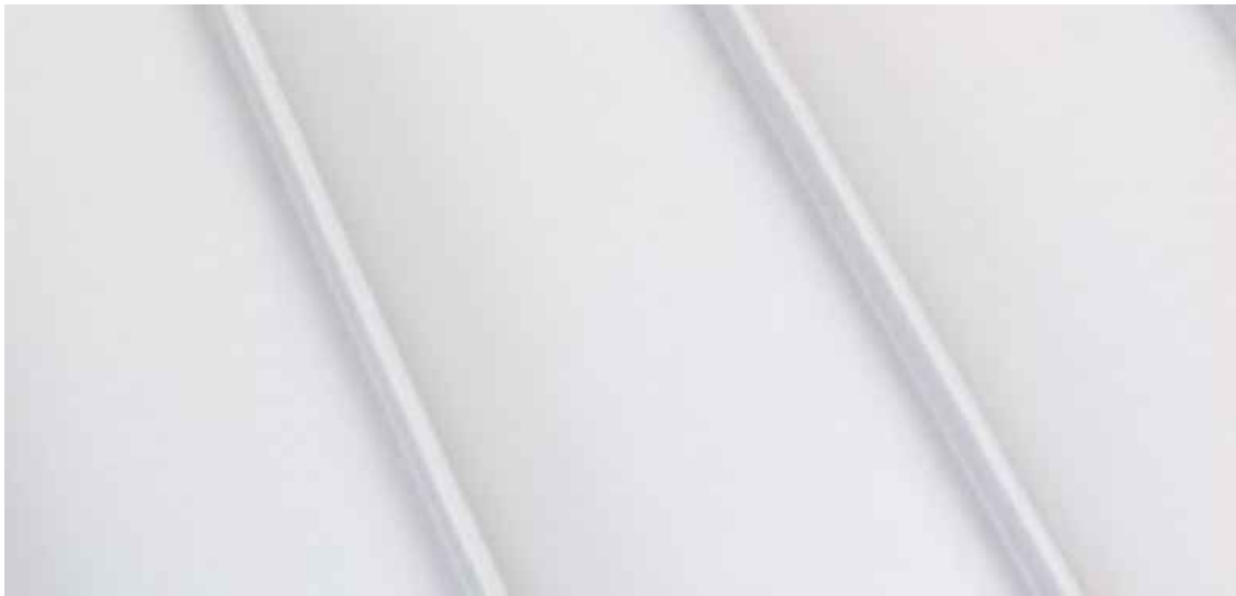
LOW SLOPE ROOF
