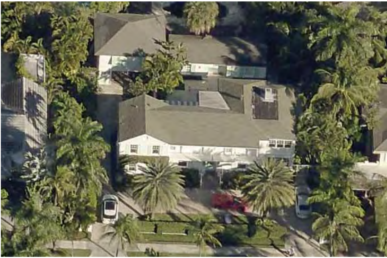
South Aerial View
