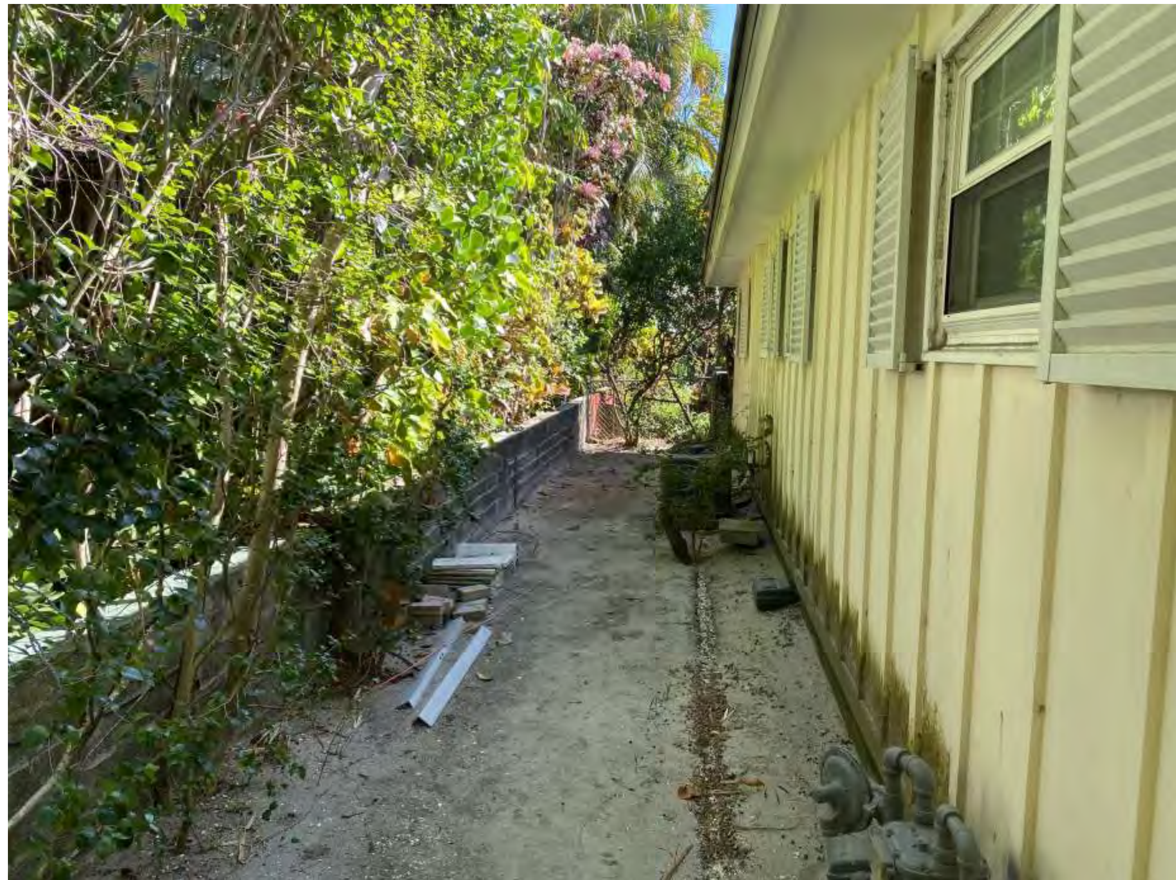
K L-5 EXISTING NORTH SIDE YARD
