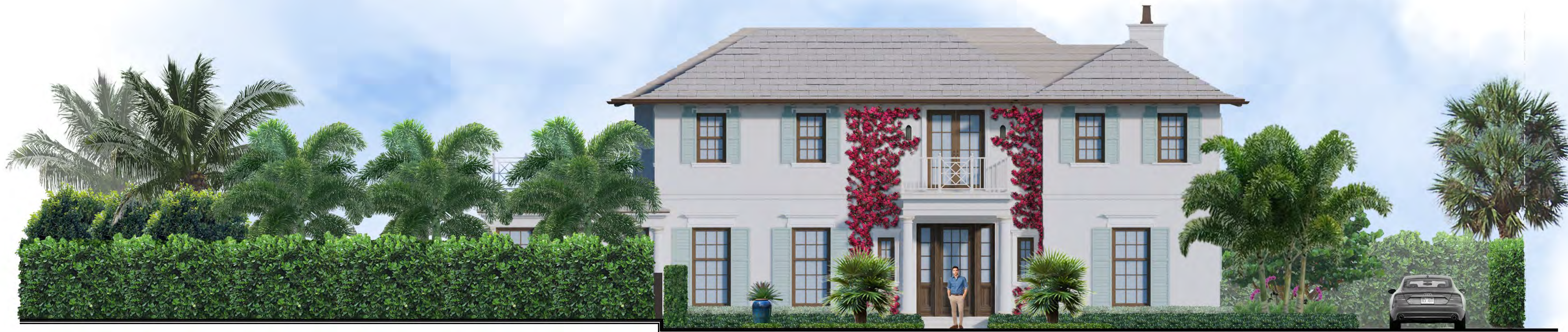
Front Elevation - Interior View
