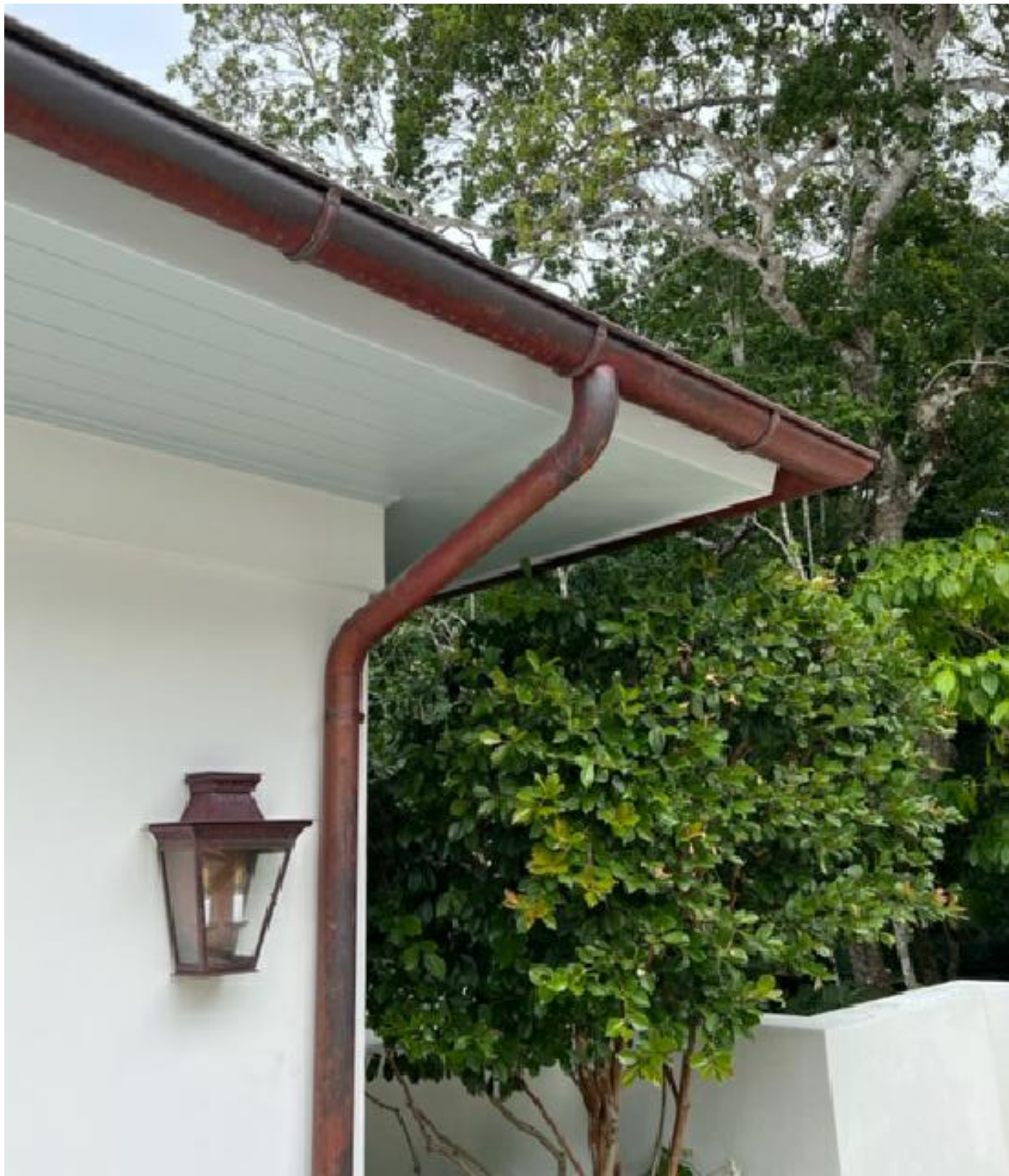
GUTTERS AND DOWNSPOUTS COPPER
