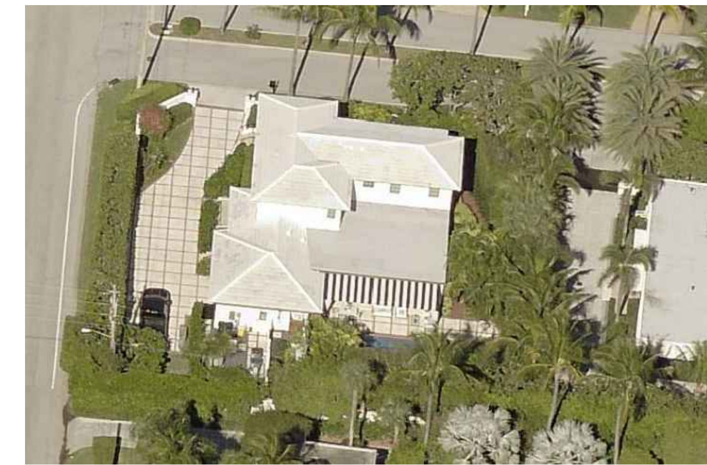
South West Aerial View
