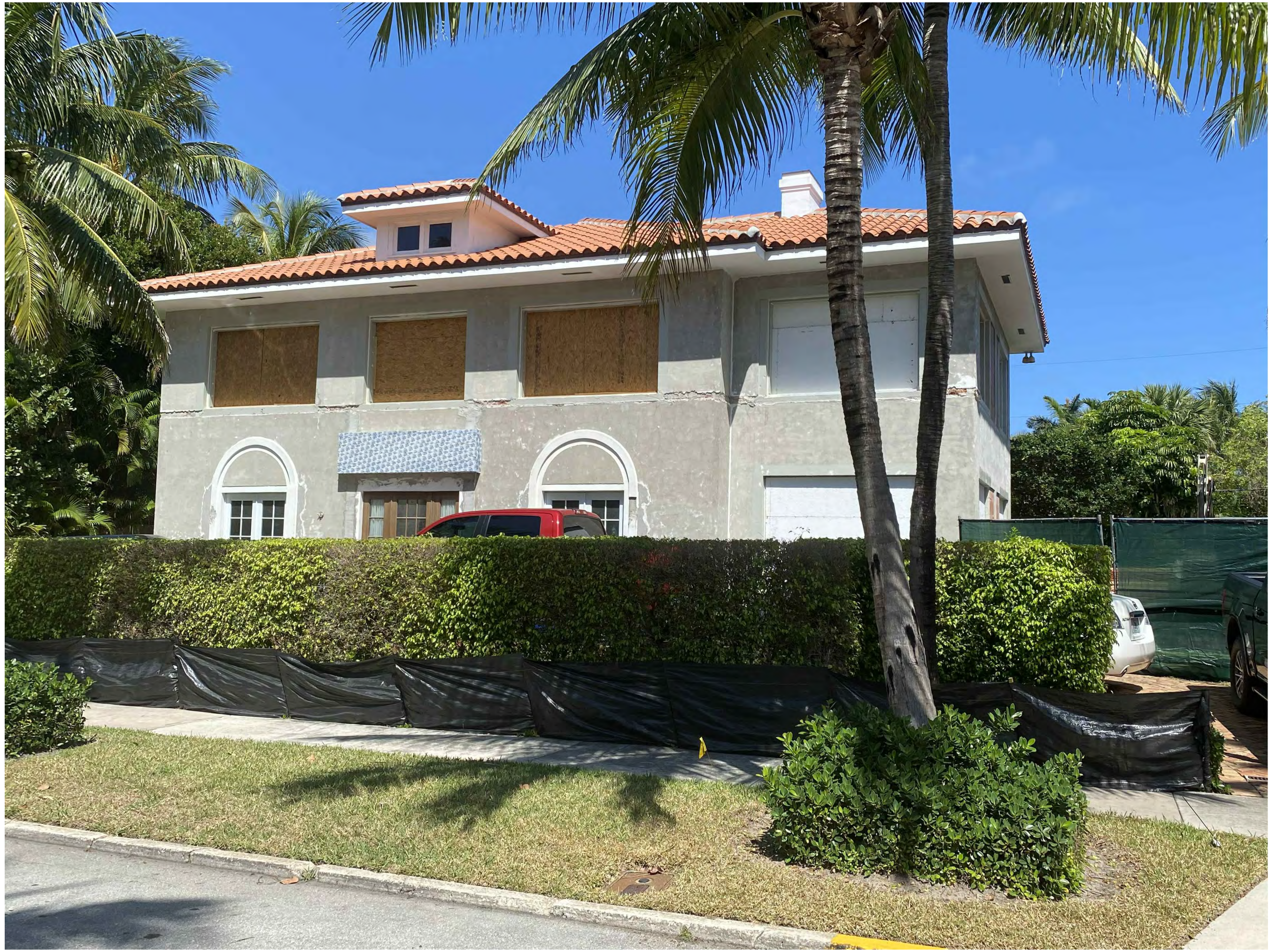
135 NORTH OCEAN BLVD (UNDER CONSTRUCTION)
