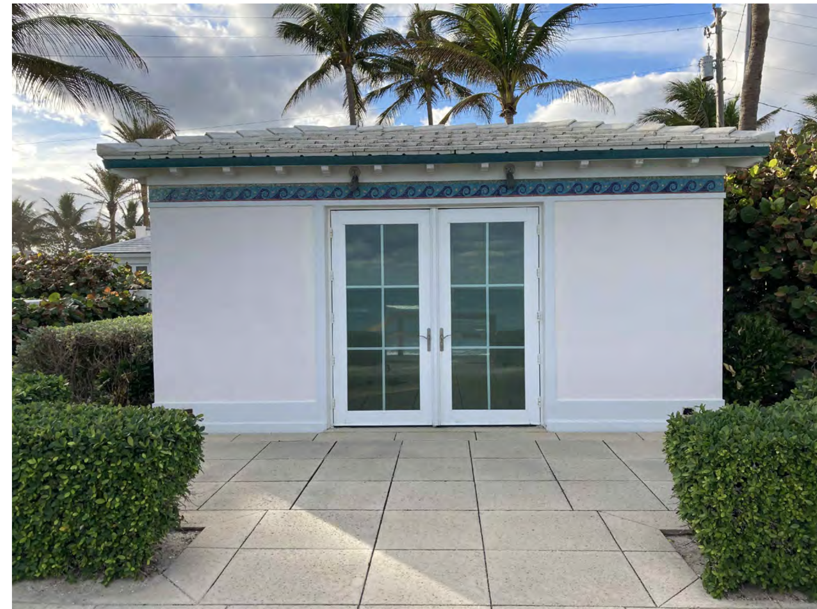
EXISTING STRUCTURE - FACING WEST
