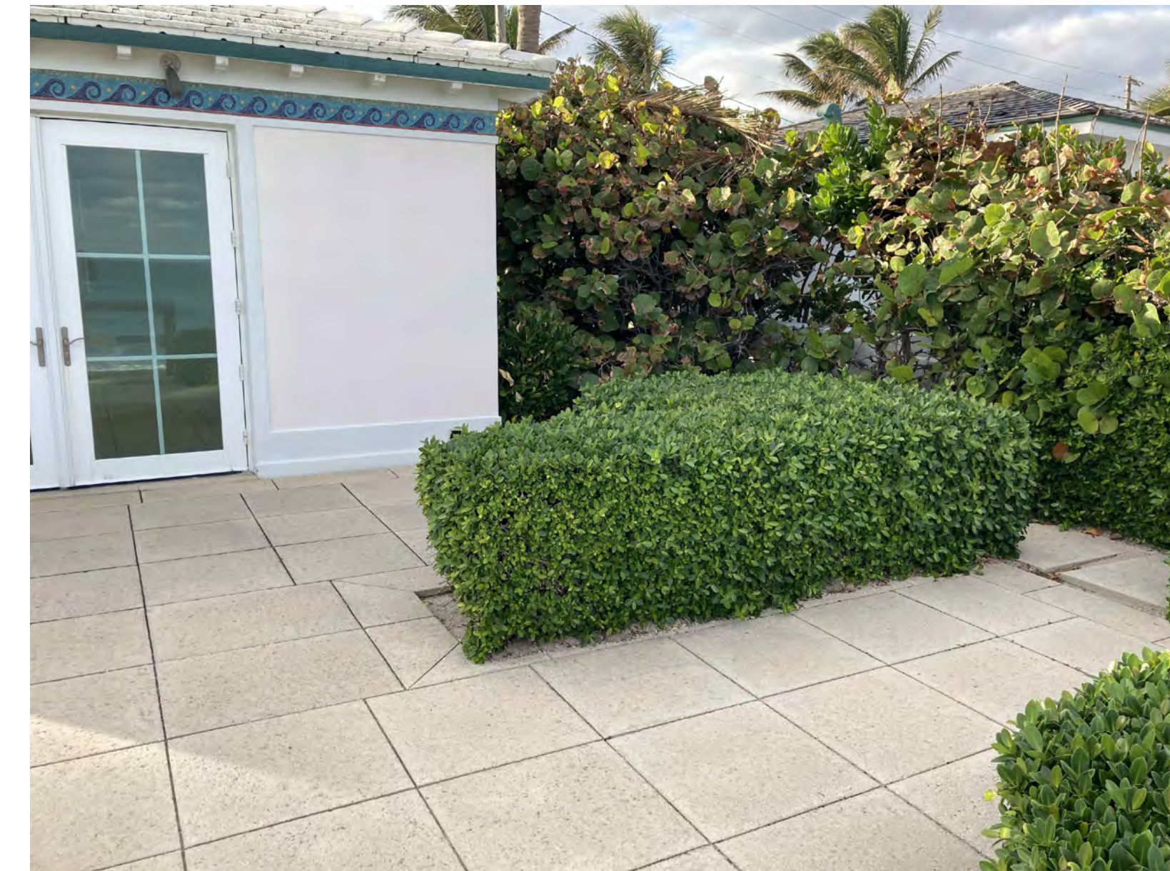
EXISTING VEGETATION & STRUCTURE - FACING NORTHEAST
