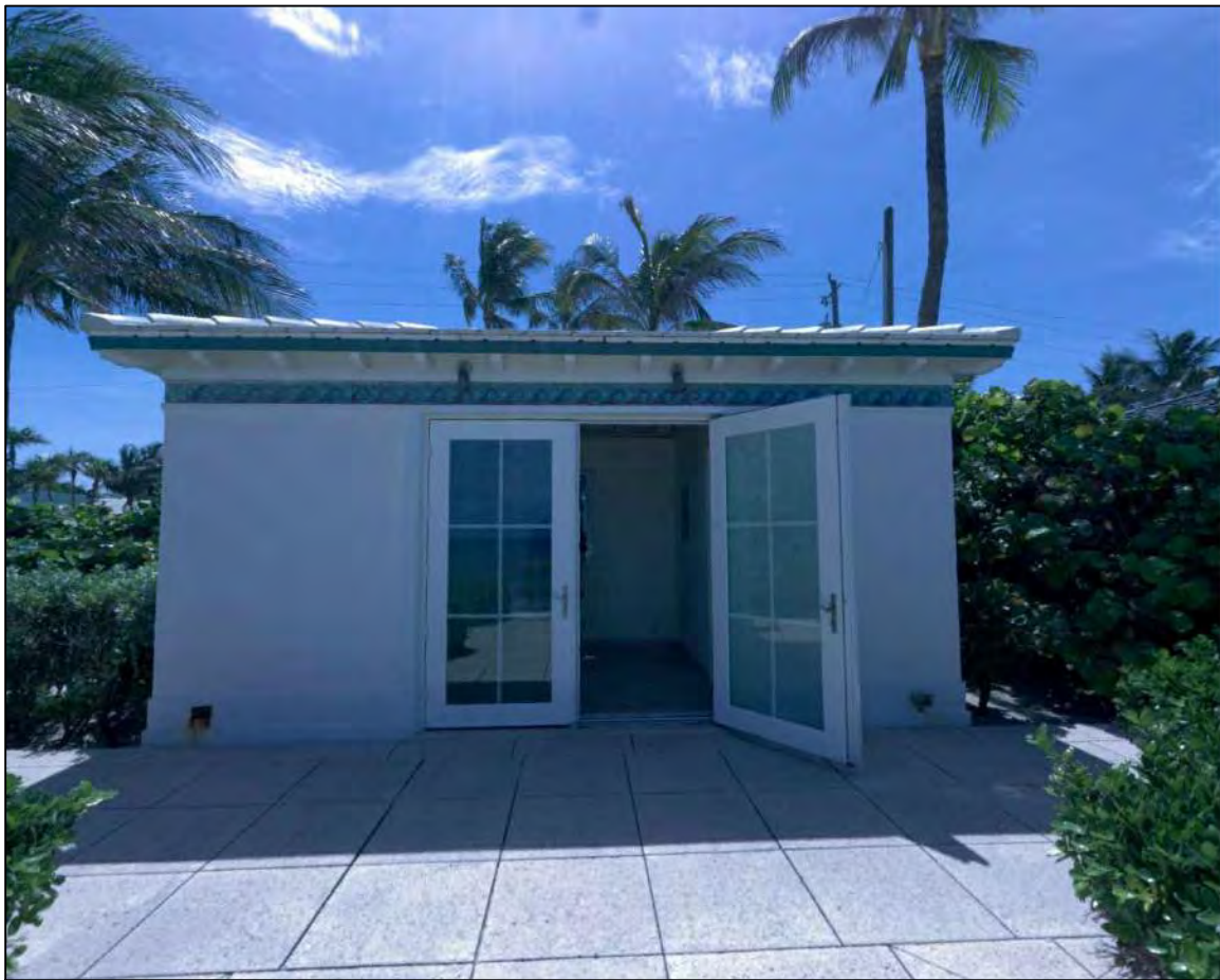
VIEW A - EXISTING CABANA ENTRANCE
