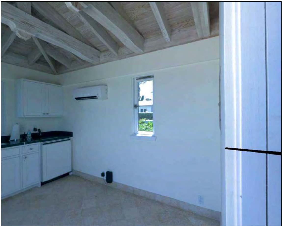
VIEW B - VIEW INTO BEACH CABANA EXISTING MILLWORK
