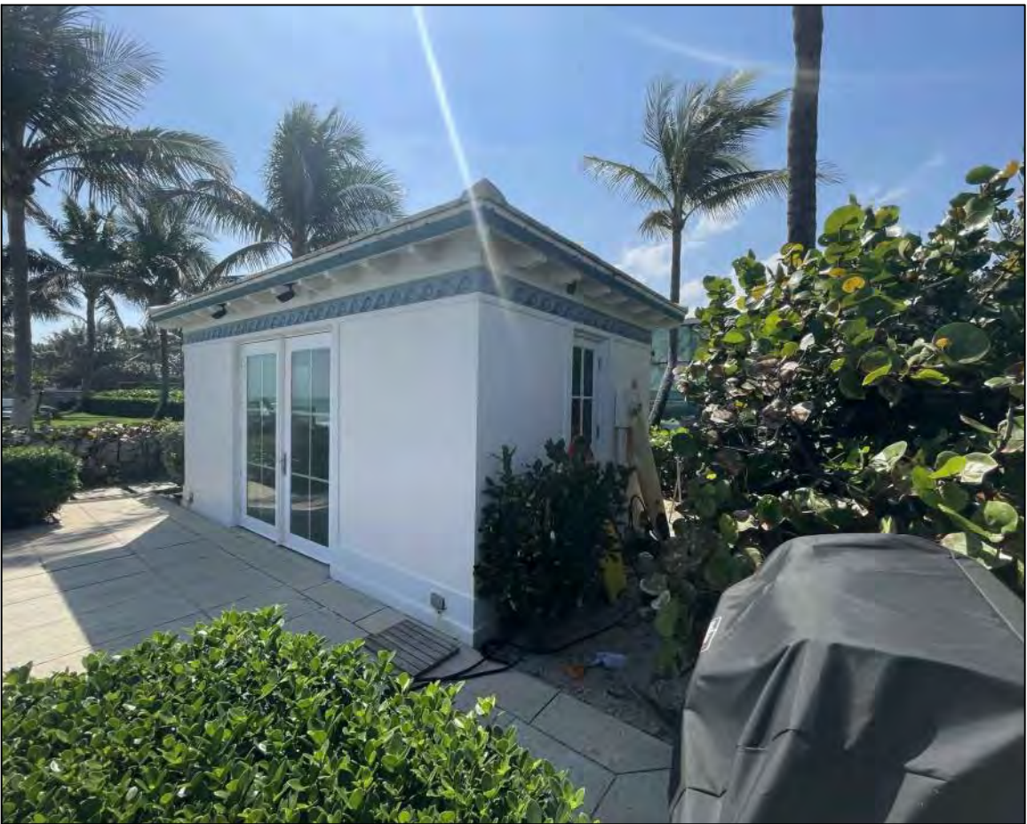
VIEW C - VIEW OF NORTH AND EAST ELEVATION
