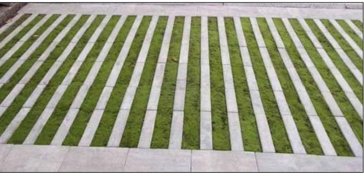
- NEW DRIVEWAY PARKING AREA LINEAR CONCRETE PAVERS W/ LAWN JOINTS
