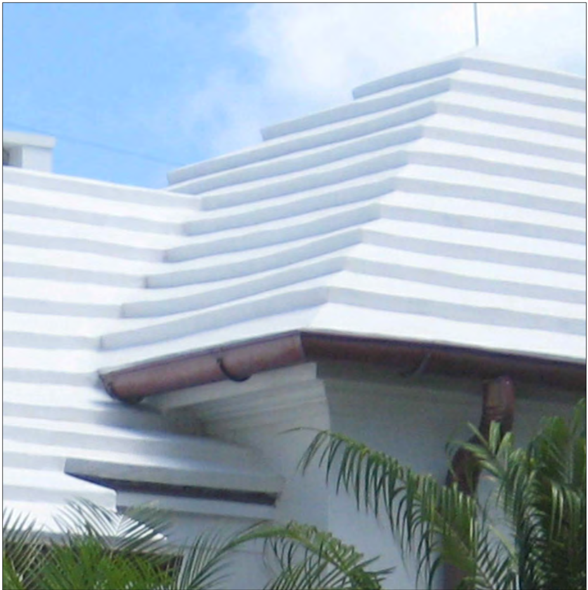
CONCRETE TILE ROOF W/ COPPER GUTTERS
