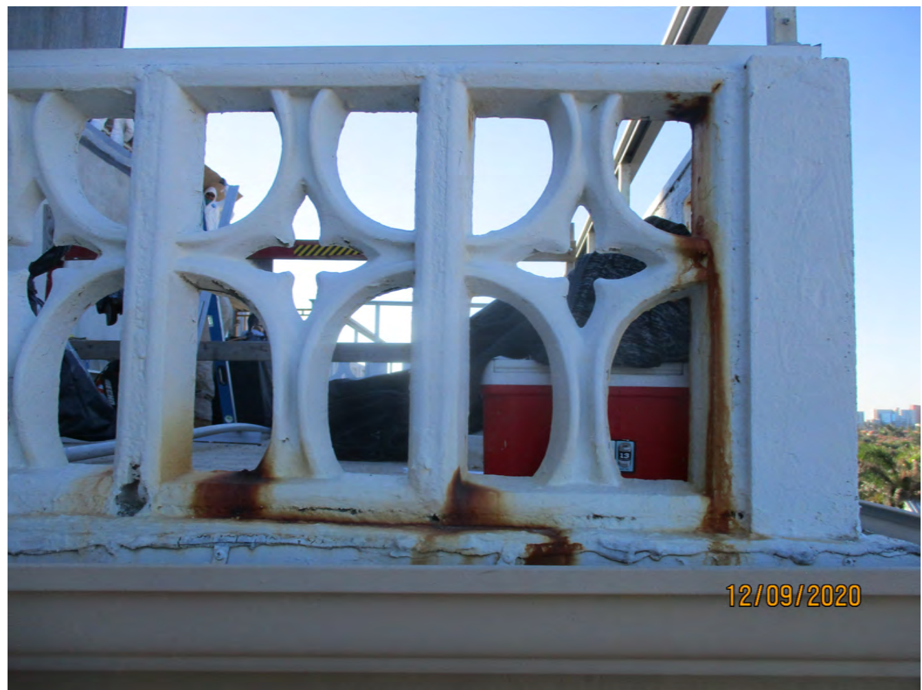
EXISTING BALCONY RAIL TO BE REPLACED
