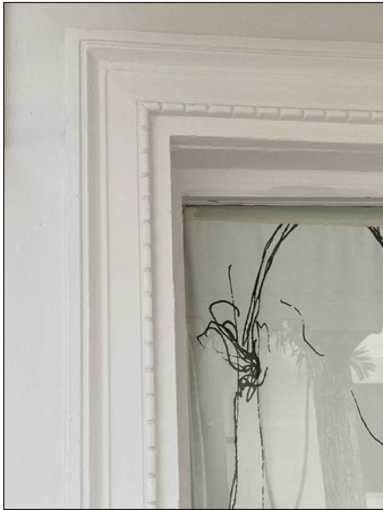
Existing / Proposed /stepped Plaster Moulding Detail (typical for all existing / new doors)
