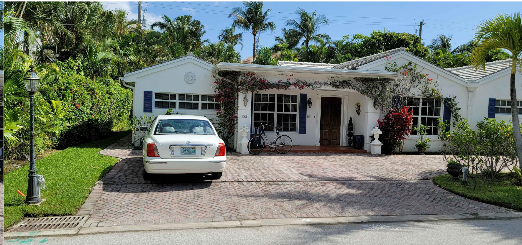
1 2.5 249 FAIRVIEW ROAD - SOUTH FACADE
