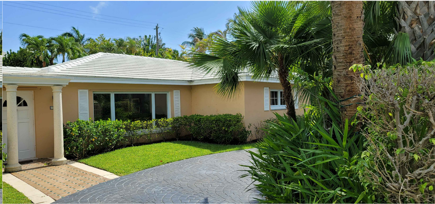
4 2.5 257 FAIRVIEW ROAD - SOUTH FACADE
