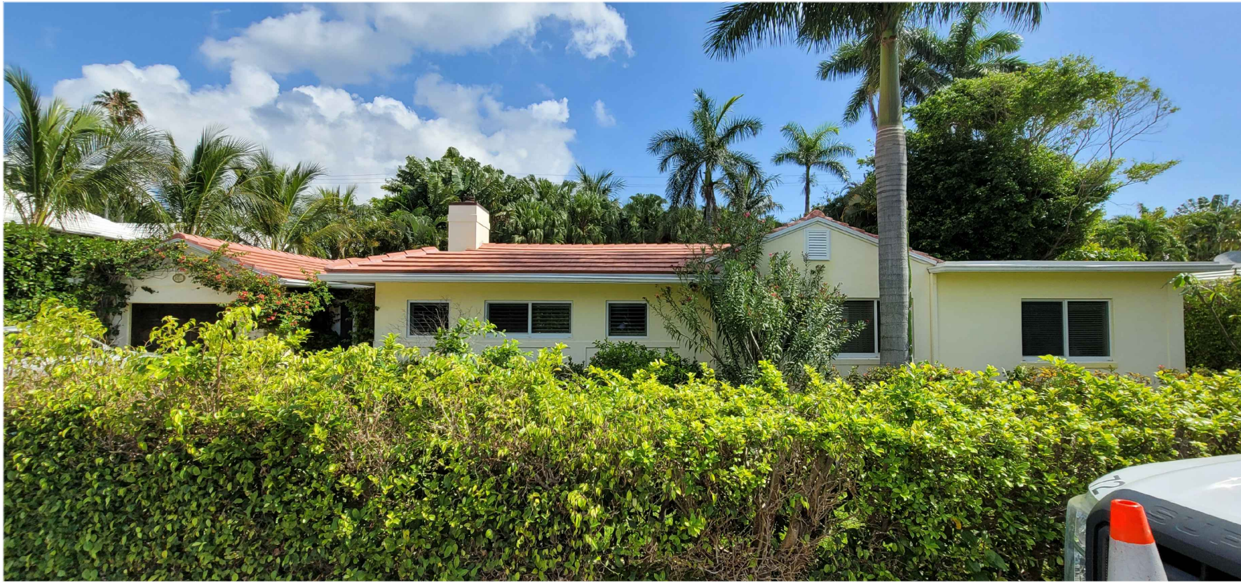
6 2.5 265 FAIRVIEW ROAD - SOUTH FACADE
