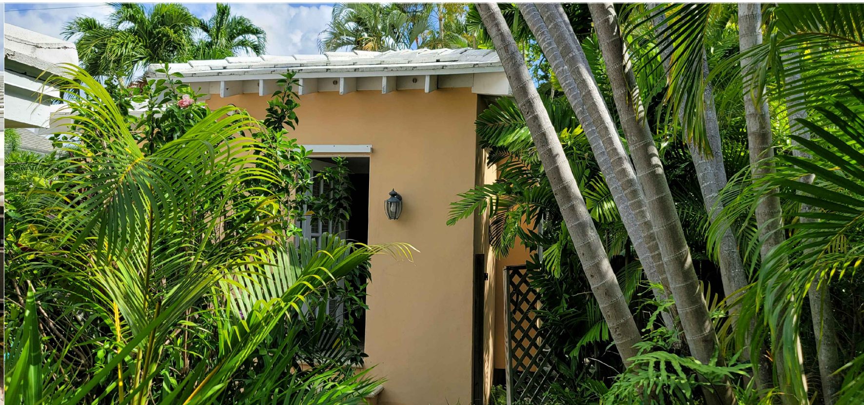
8 2.5 257 FAIRVIEW ROAD - POOL HOUSE S. FACADE
