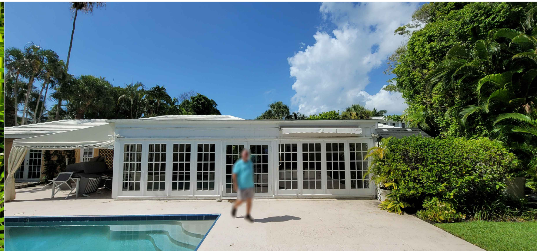
11 2.5 257 FAIRVIEW ROAD - NORTH FACADE
