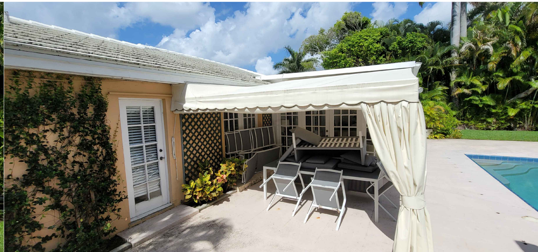
10 2.5 249 FAIRVIEW ROAD - LANAI NE FACADE
