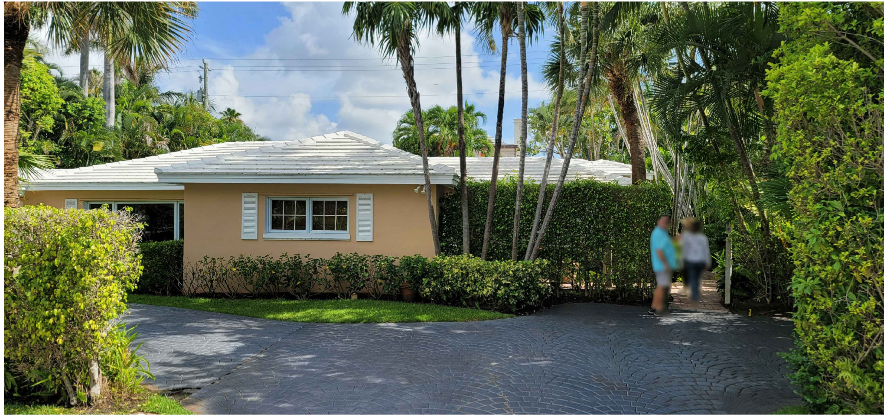
3 2.5 257 FAIRVIEW ROAD - SOUTH FACADE
