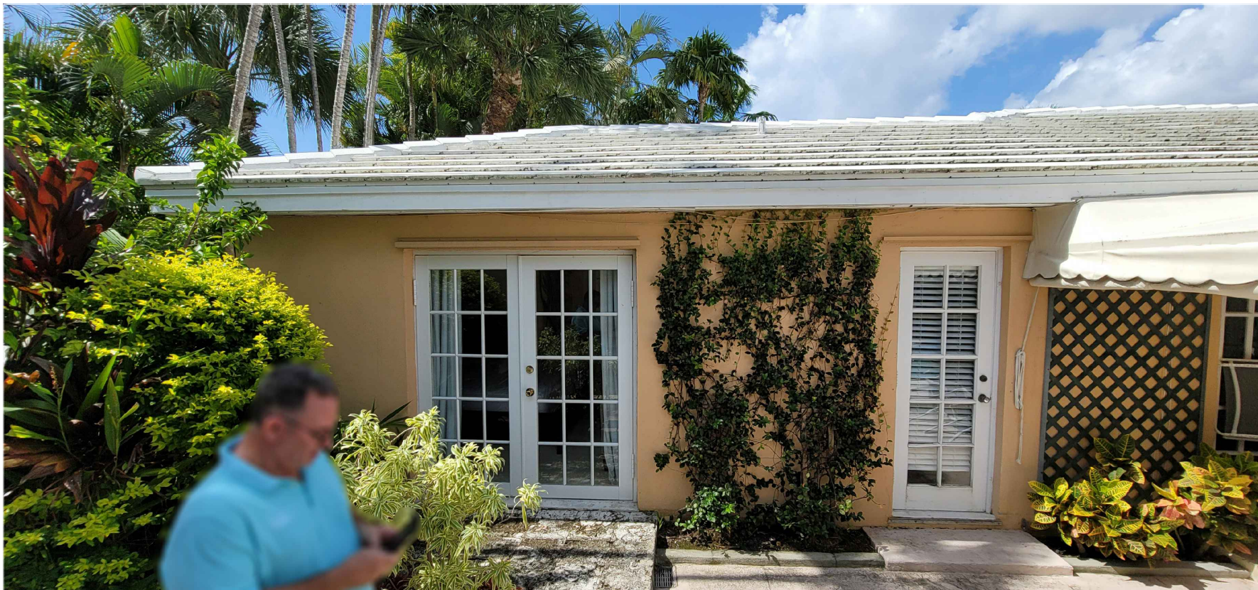
9 2.5 257 FAIRVIEW ROAD - NORTH FACADE
