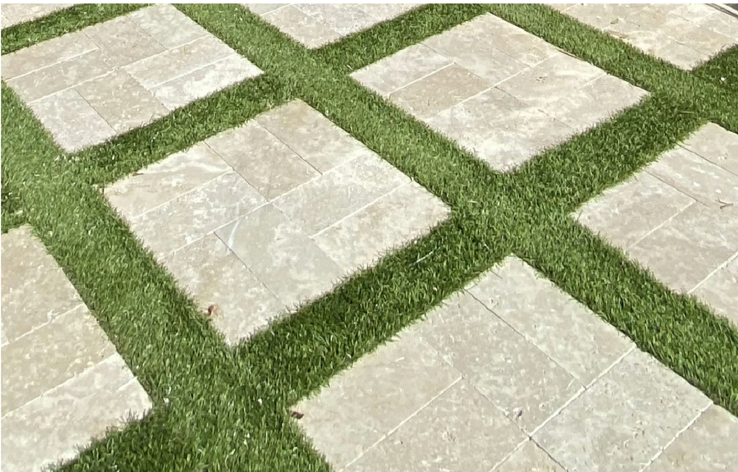
EXISTING CONDITION: ARTIFICIAL TURF JOINTS
