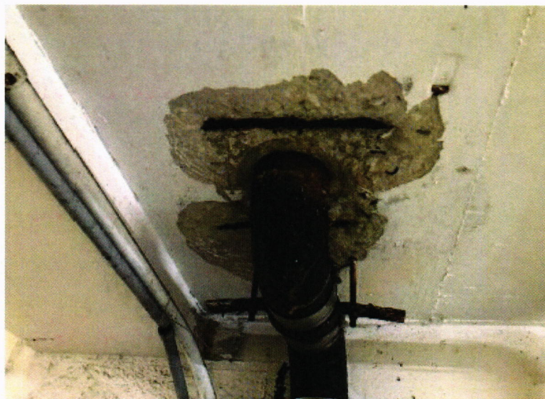
Figure 14 – Delaminating concrete and exposed reinforcement at elevated slab. Repair Type A required.
