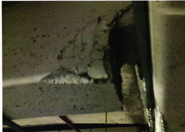
Figure 11 – Concrete spalling at precast beam. Repair Type A required.
