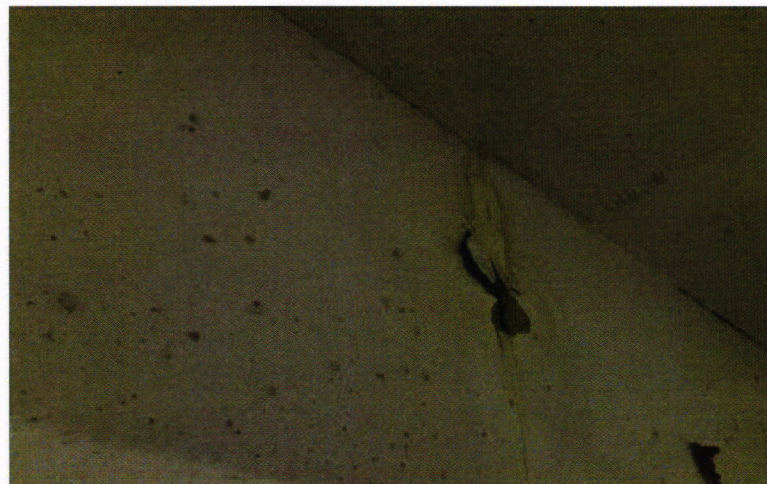
Figure 17 – Exposed rebar and spalling concrete on precast joist. Condition as seen during the 9/24/2021 site visit. Repair Type A required.
