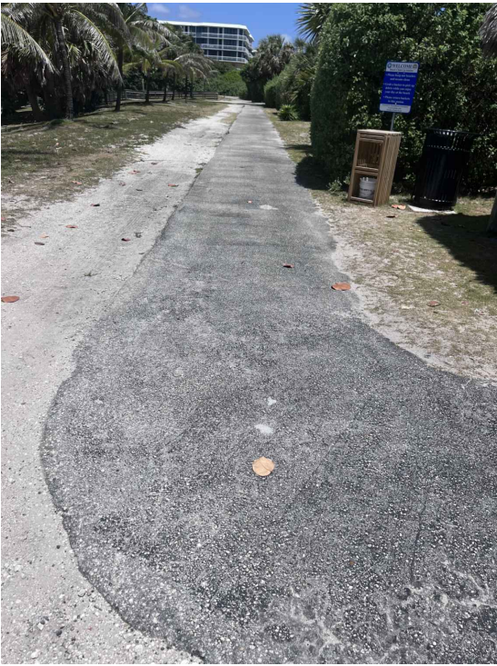
PICTURE 22: SHELLROCK AND ASPHALT PATH
