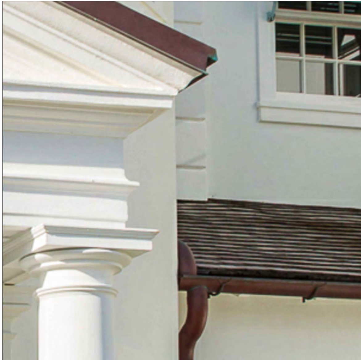
FLASHING, DOWNSPOUTS, & GUTTERS COPPER
