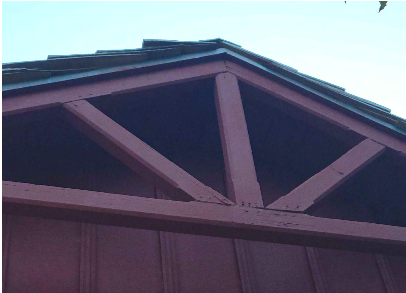
2 WEST ELEVATION GABLE TRUSS
