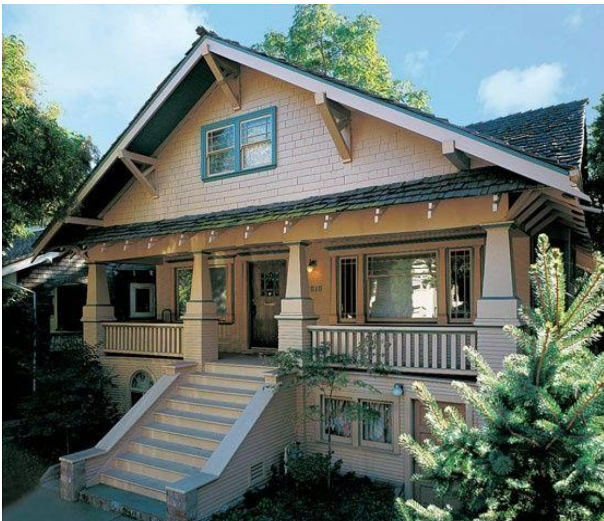
Outlookers and brick to shake transition
