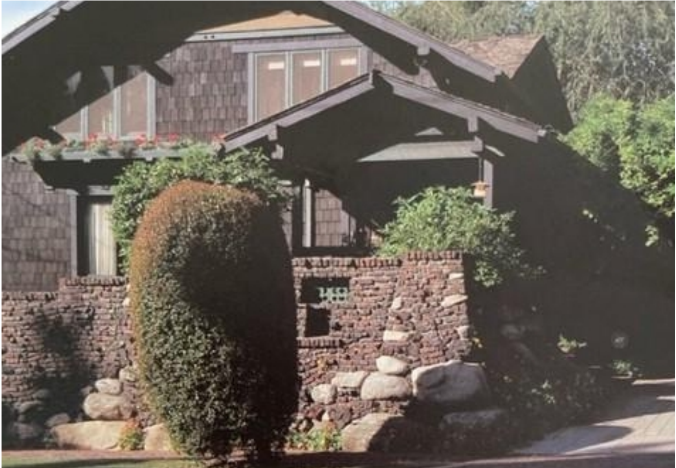
Tapered stone & brick base - Van Rosem-Neill House
