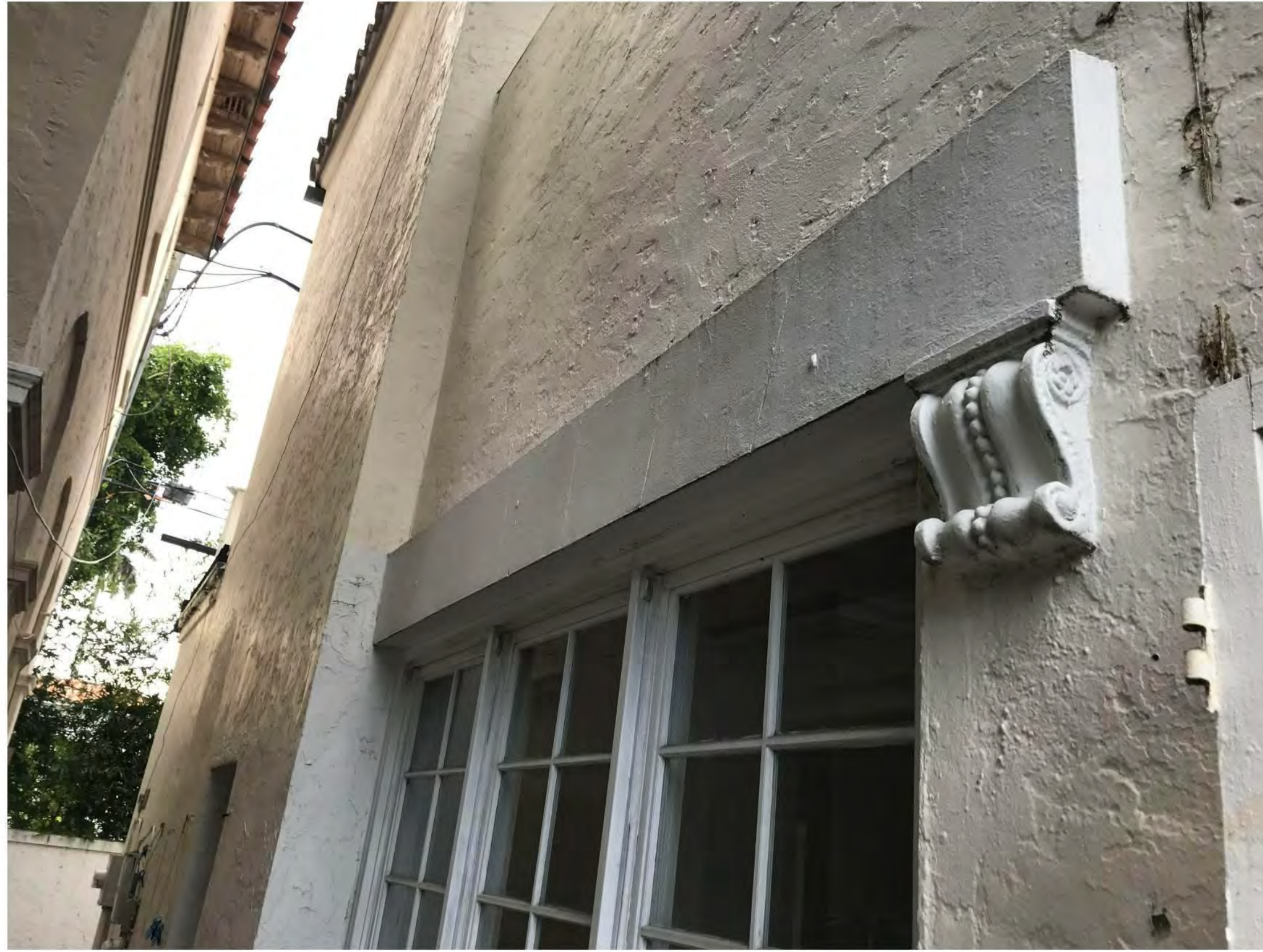
2 EXISTING CAST STONE LINTEL AND CORBEL
