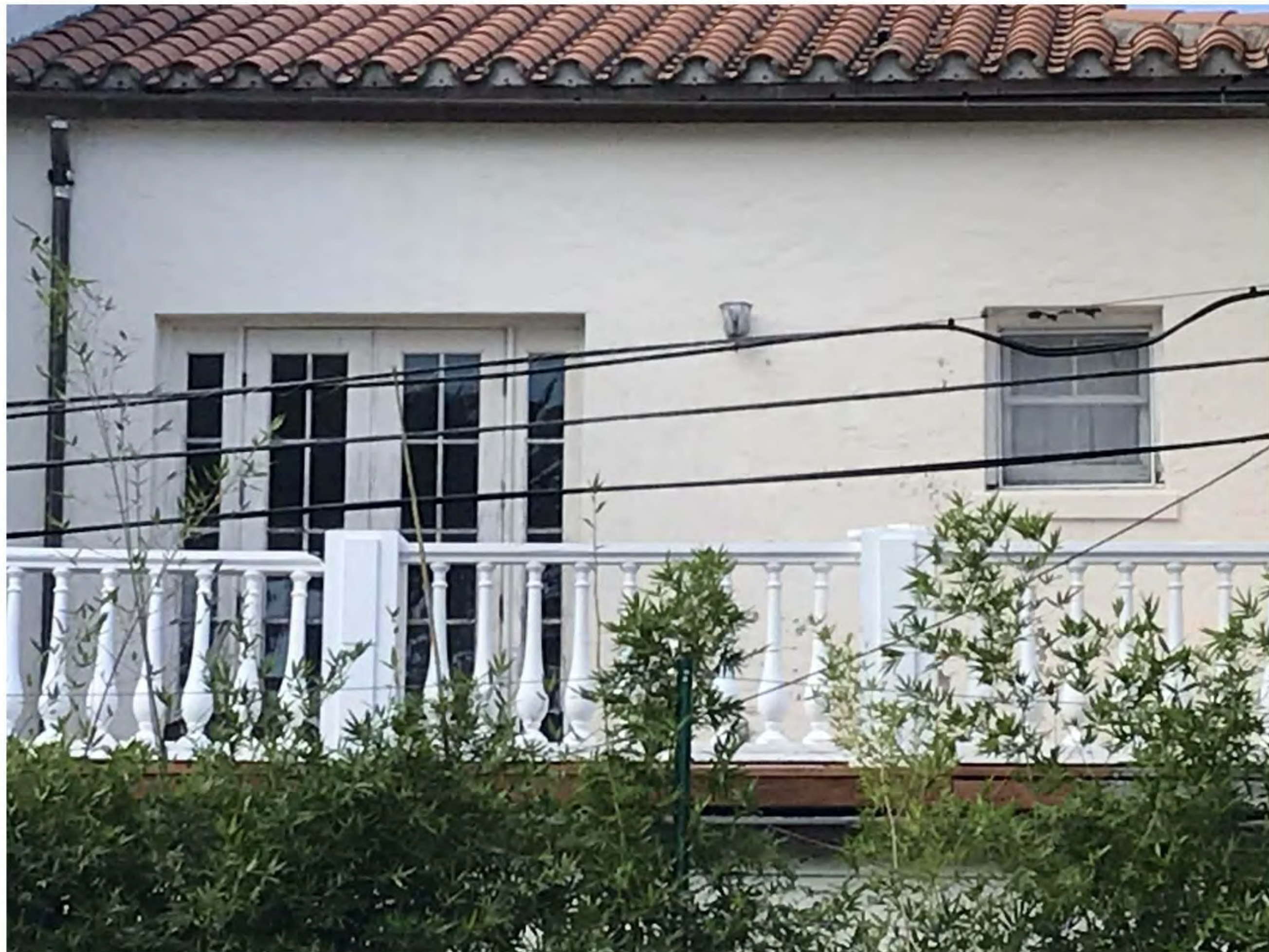
4 EXISTING CAST STONE RAILING
