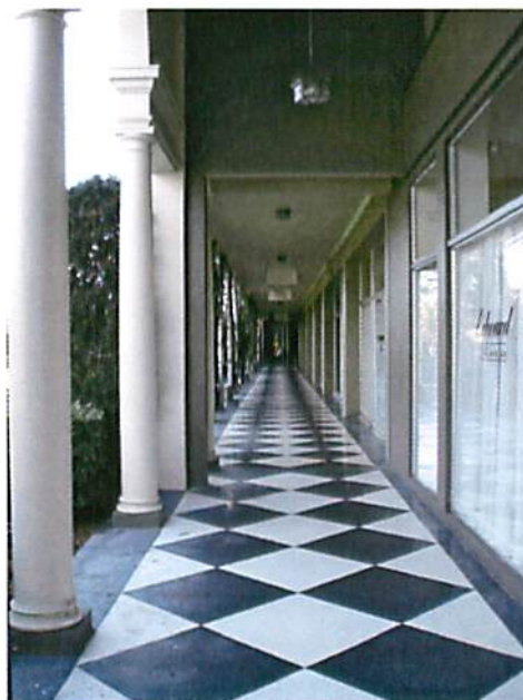
Polished black and white terrazzo flooring enhances the covered walkways at the Shopping Plaza.
