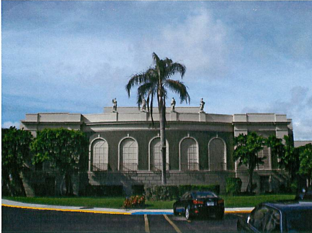
The east facade of the Royal Poinciana Playhouse.
