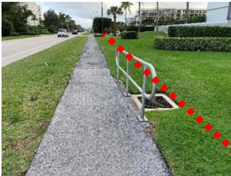
FDOT Catchbasin in front of 2860 South Ocean Blvd
