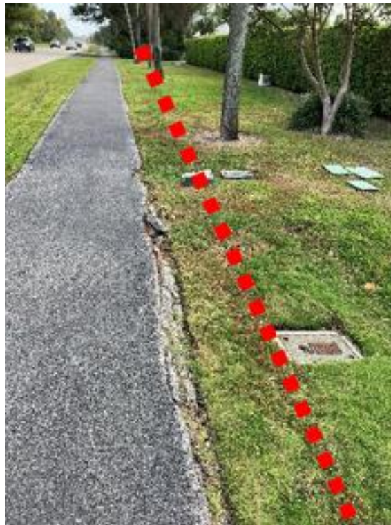
Existing Water Meter and Irrigation Valve Boxes
