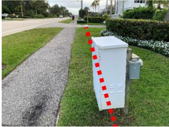
Existing Communications Utility Panel
