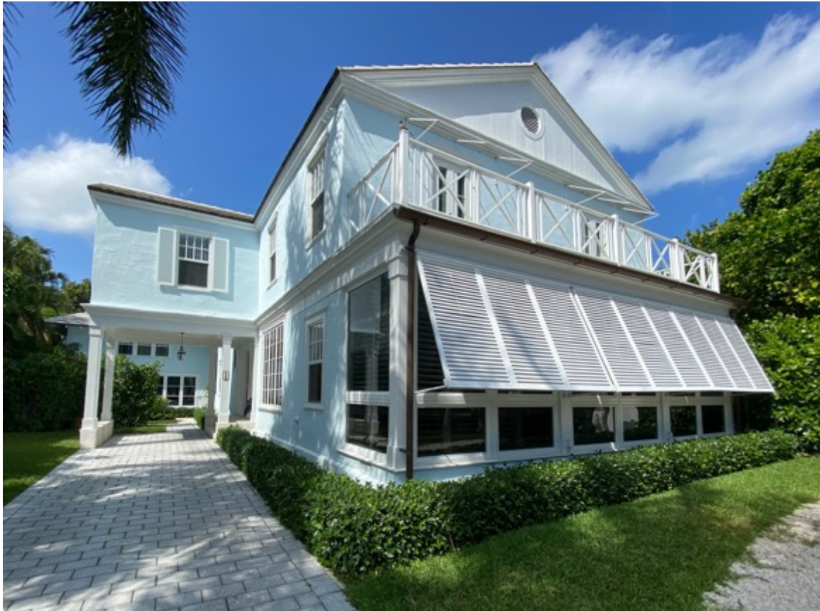
South and West Facades Looking Northwest
