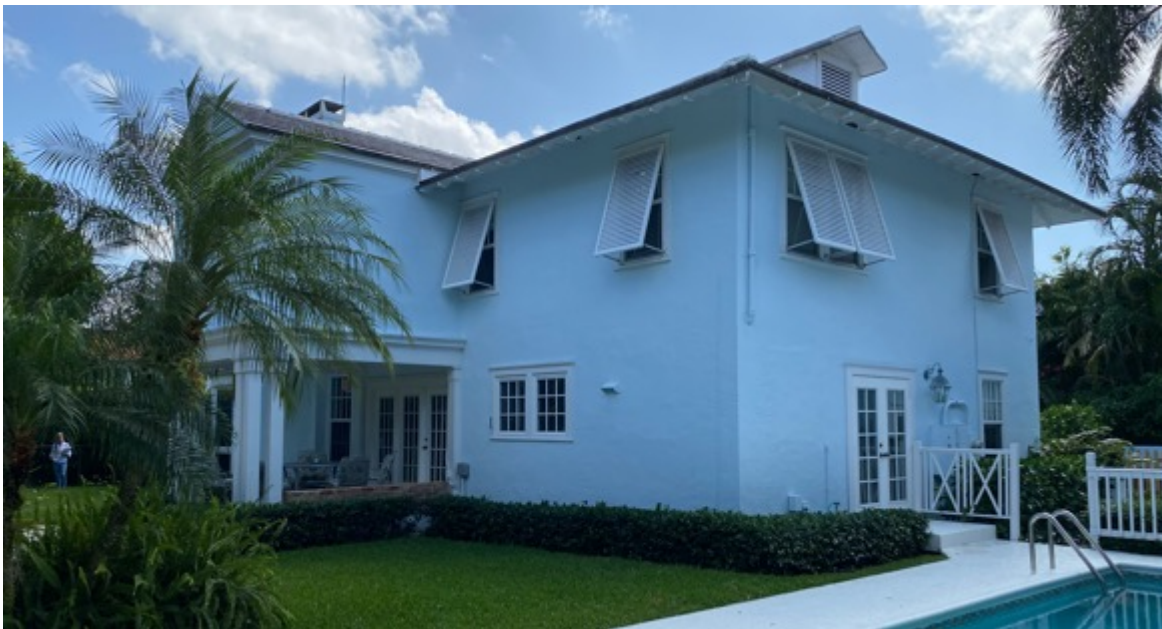
East and North (Rear) Facades Looking Southwest
