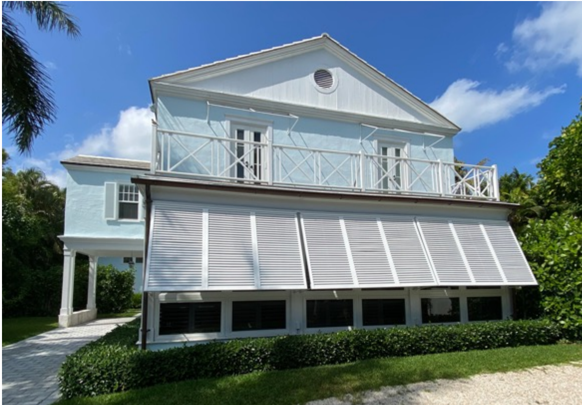
South Façade Looking North
