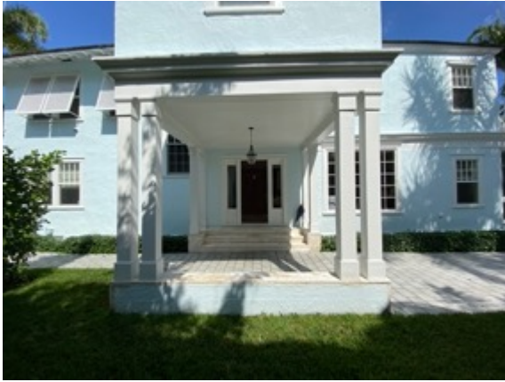
West Façade Entry to Dwelling Looking East.
