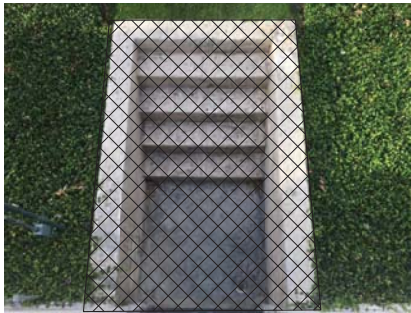
PUMP ROOM STAIR REMOVAL SCALE: NTS
