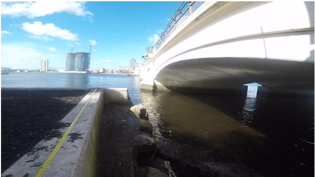
Figure 3.8: Sta 0+02 looking west. Corrugated face and offset cap.
