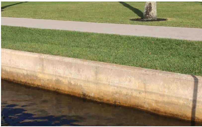
Figure 8.4: Bulkhead Fronting the Town Docks
