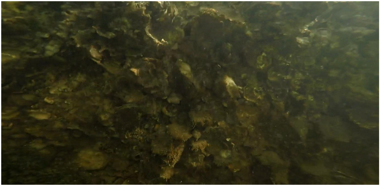
Figure 3.5: Typical marine growth on the concrete face of the bulkhead.
