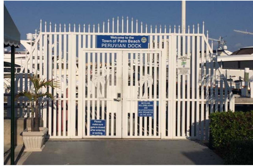
Figure 6.2: Gate and Keypad at Peruvian Dock
