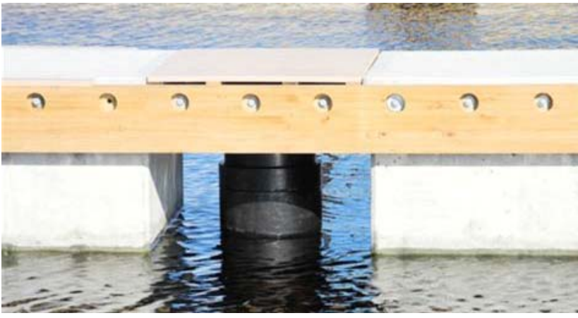
Figure 4.1: Dock with a Telescoping Pile (Bellingham)
