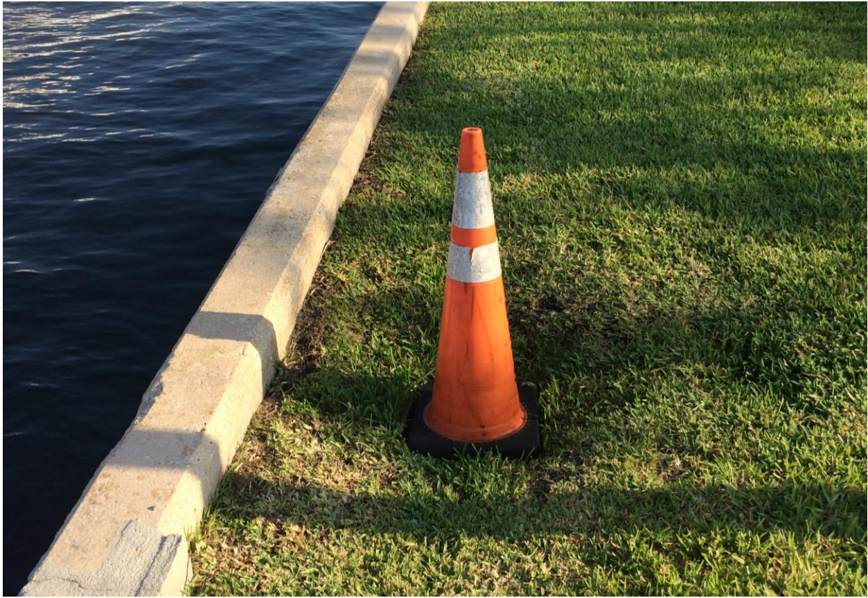
Figure 3.17: Sta 10+80. Area with backfill loss.
