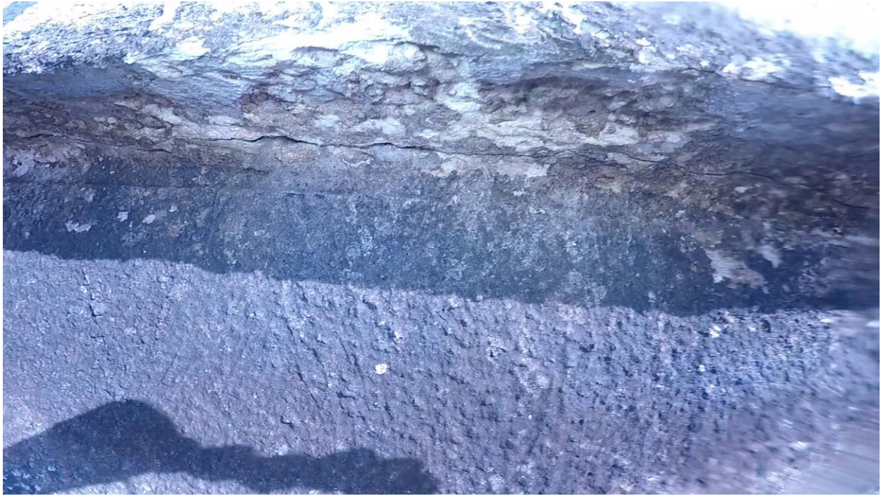
Figure 3.13: Sta 15+00. Cracking, spalling and deterioration underneath the lip along the parapet bulkhead section.
