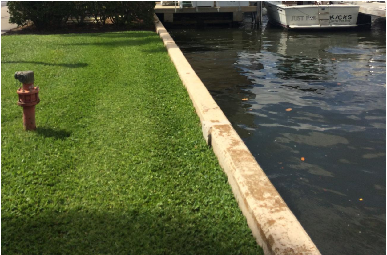
Figure 3.1: Sta 8+00 looking south. View of backfill close to the bulkhead cap elevation.
