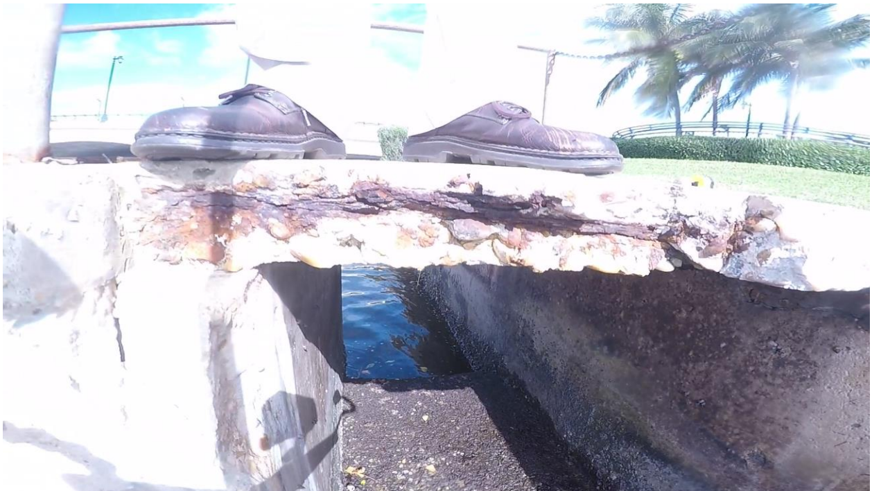
Figure 3.15: Sta 0+88 looking north. Spalling and rebar exposure and corrosion of the walkway to the outfall structure.
