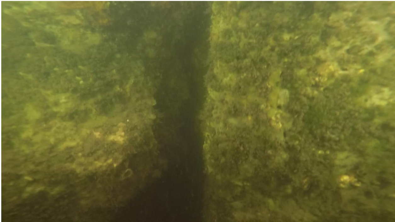
Figure 3.7: Sta 0+70. Crack at an expansion joint in the vertical concrete face.
