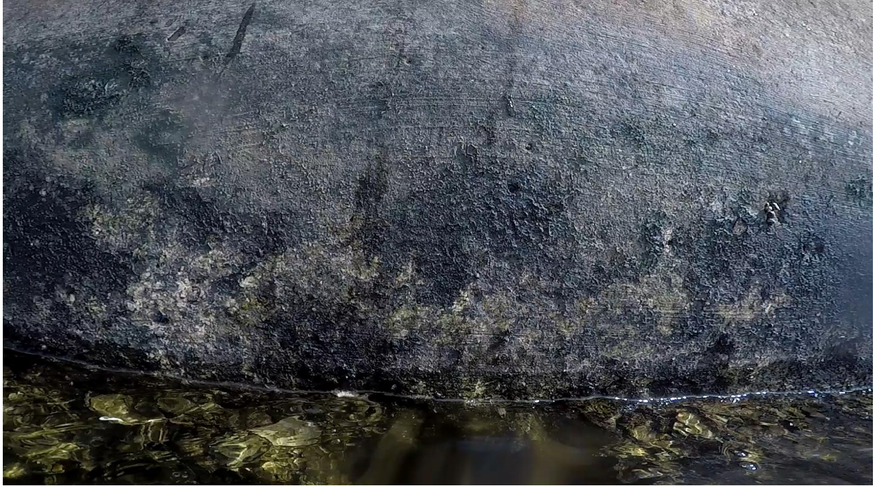
Figure 3.4: Sta 2+90. Typical bulkhead face transition from exposed concrete to the concrete covered in marine growth within in the intertidal zone.
