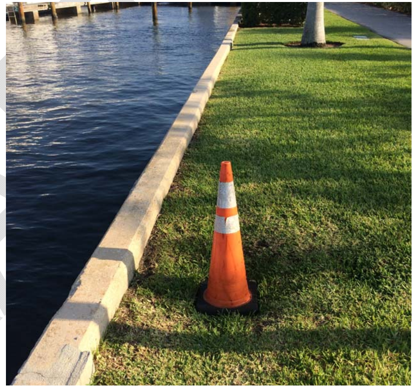
Figure 8.5: Backfill Loss behind the Bulkhead
