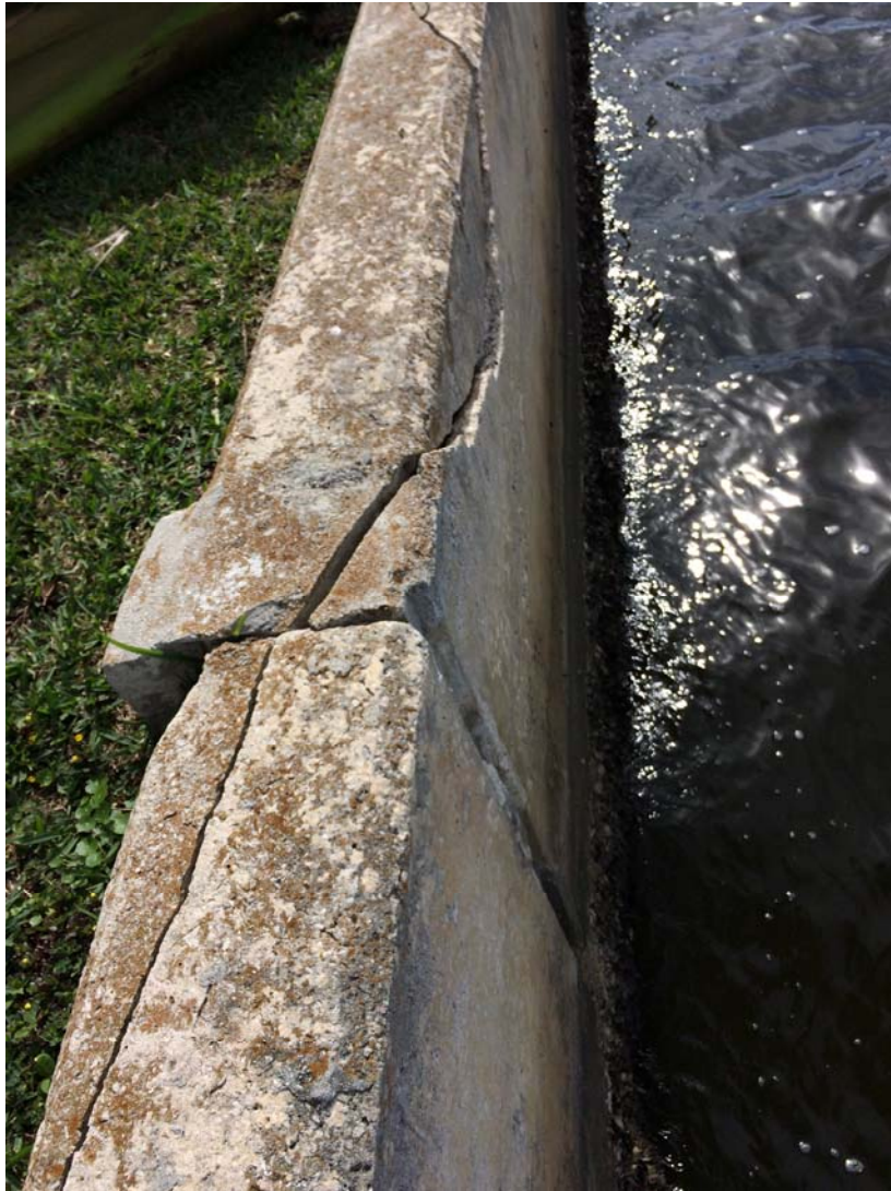
Figure 8.6: Cracking in the Bulkhead
