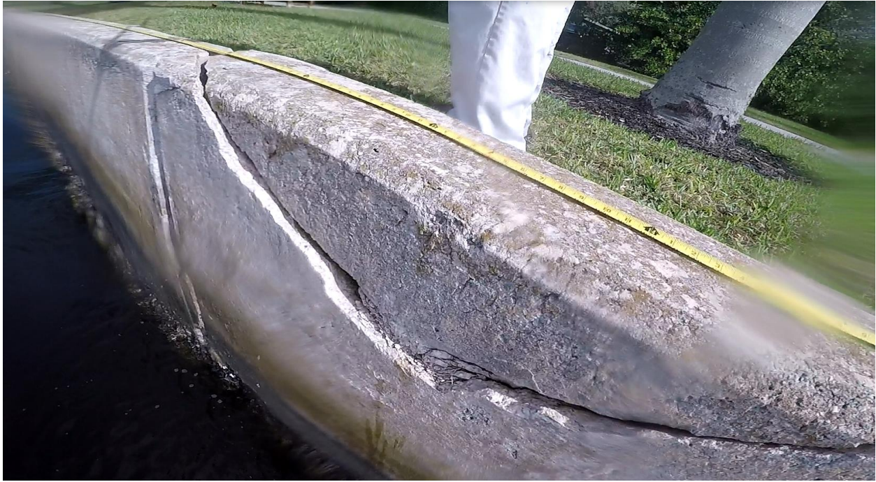
Figure 3.16: Sta 2+10. Crack and dislocated concrete cap.
