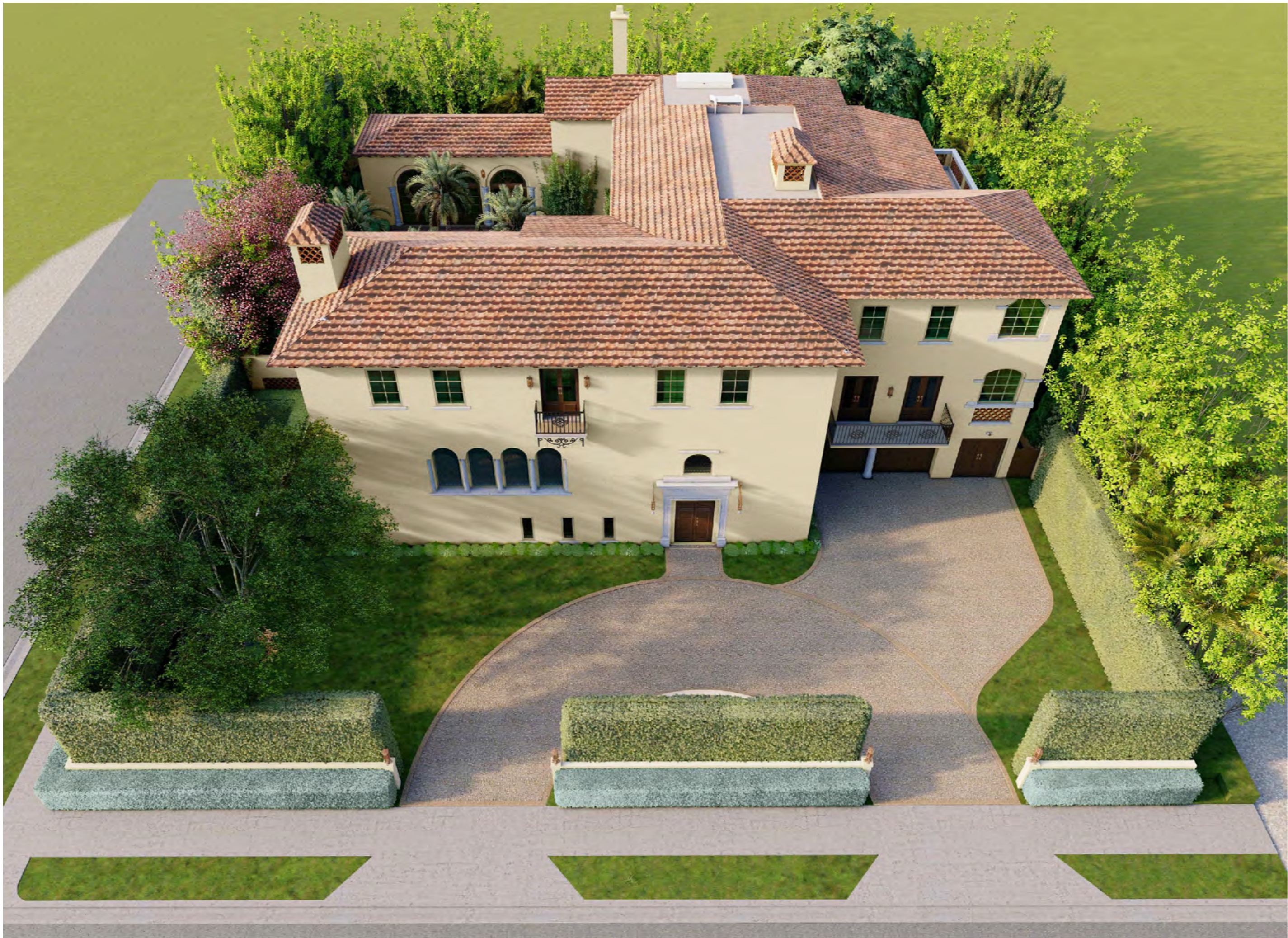
AERIAL VIEW: FRONT FAÇADE
