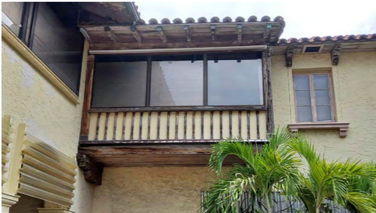
EXISTING WEST BALCONY
