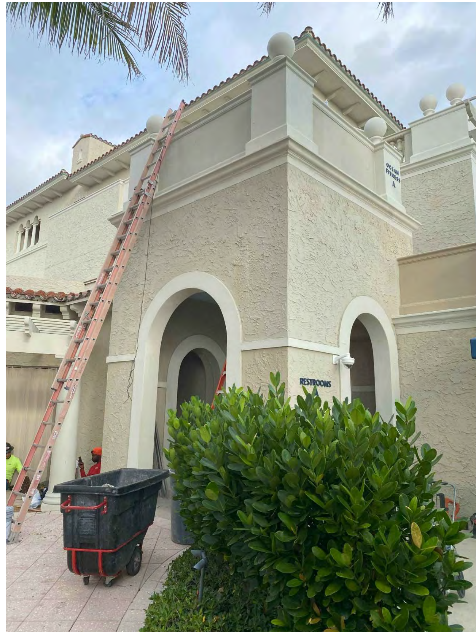
1- EXISTING RESTROOM ENTRY LOOKING NORTHWEST
