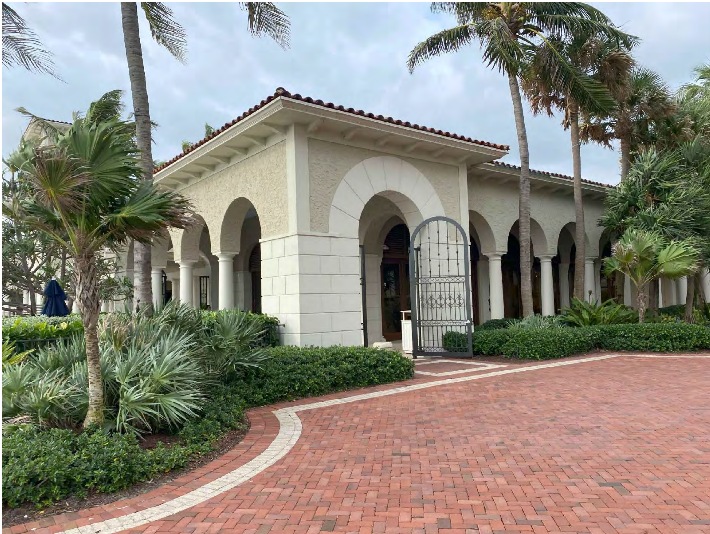
1- EXISTING SPA ARCADE ENTRY LOOKING SOUTHWEST
