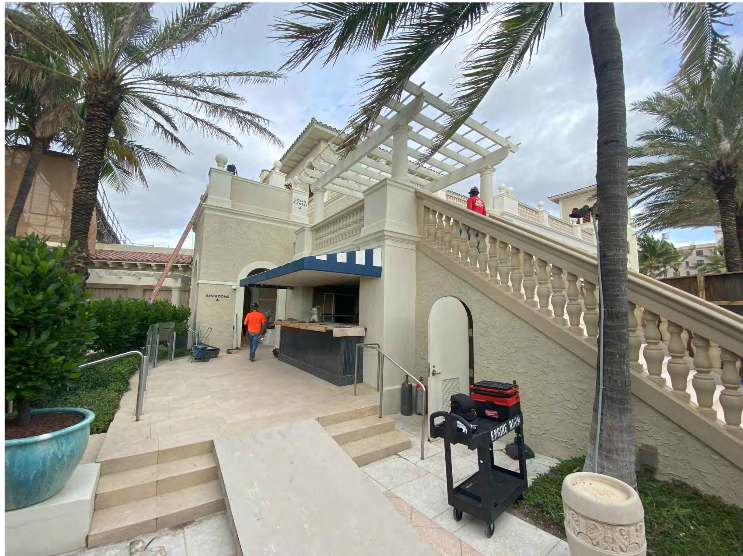
3- EXISTING OUTDOOR BAR LOOKING NORTHWEST
