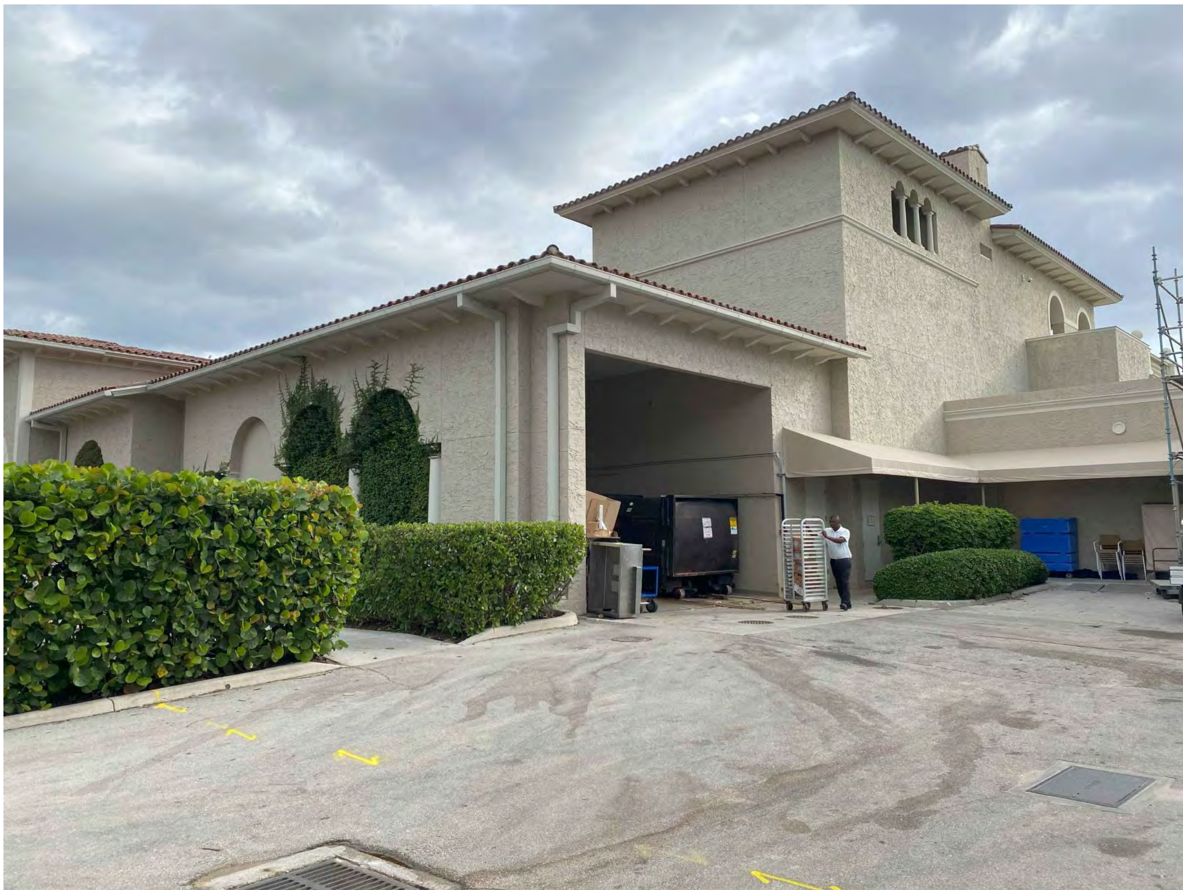
3- EXISTING LOADING ZONE LOOKING NORTHEAST
