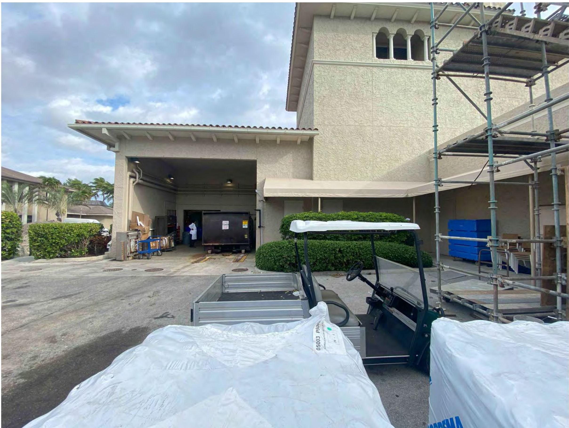
4- EXISTING LOADING ZONE LOOKING NORTH
