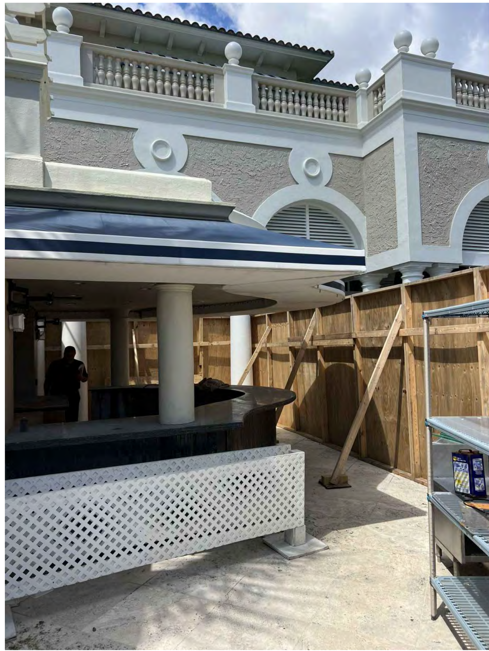
5- EXISTING OUTDOOR BAR LOOKING NORTHWEST
