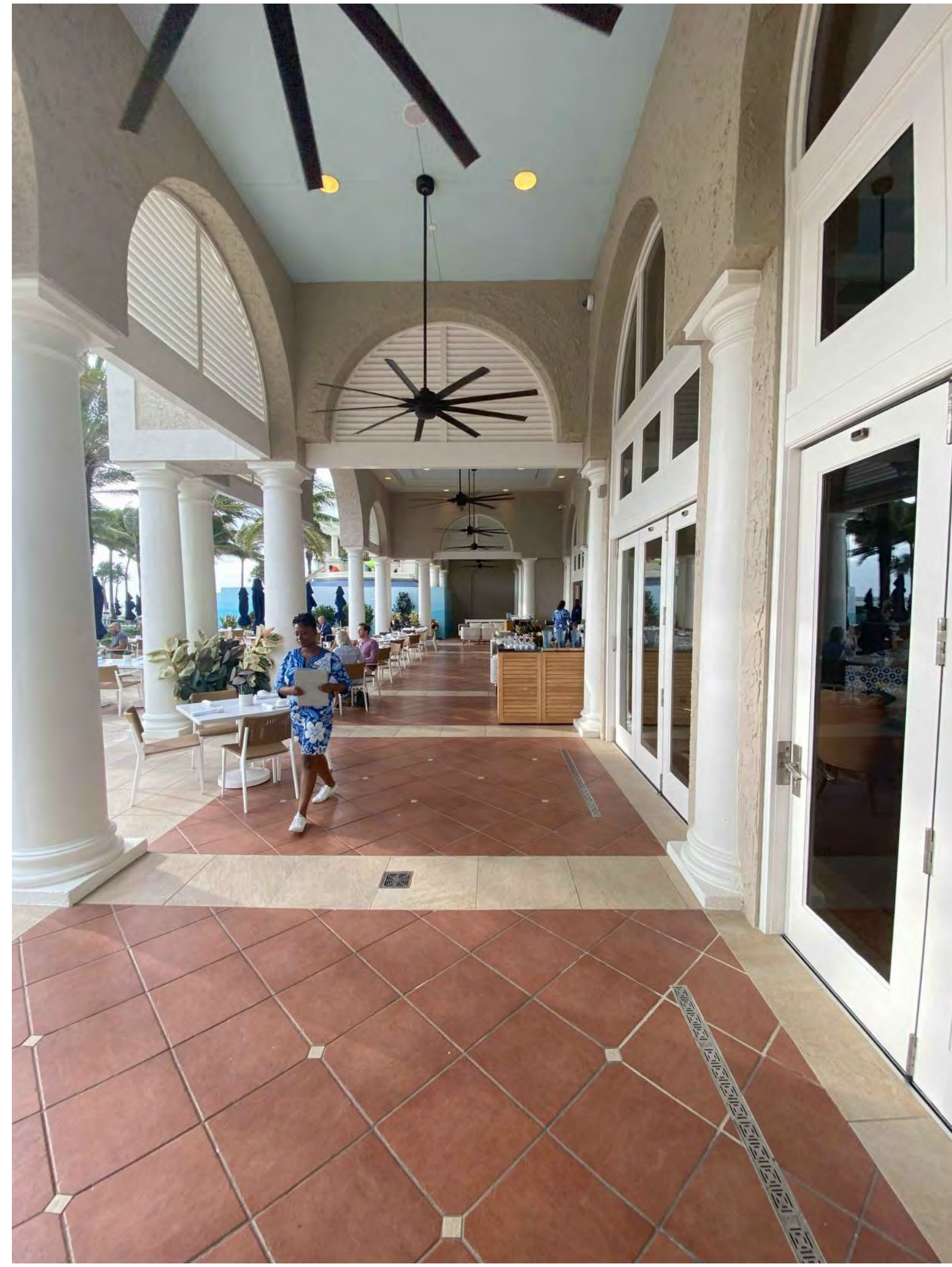
1- EXISTING LOGGIA LOOKING SOUTH
