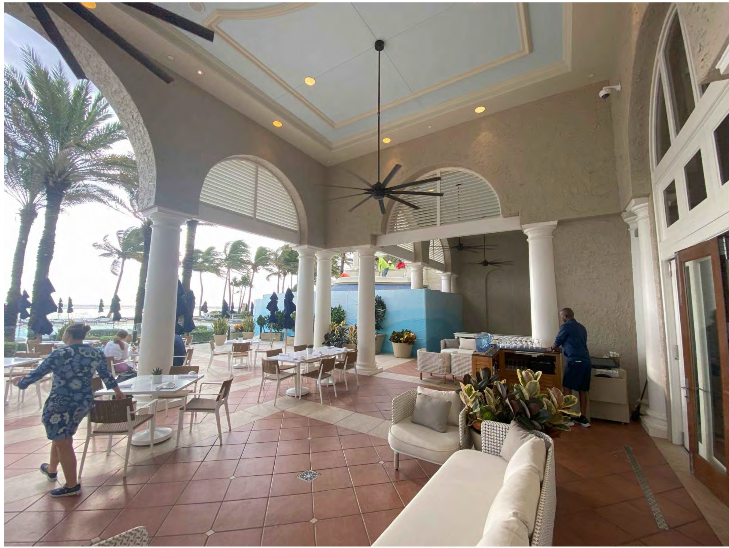
3- EXISTING LOGGIA LOOKING SOUTHEAST
