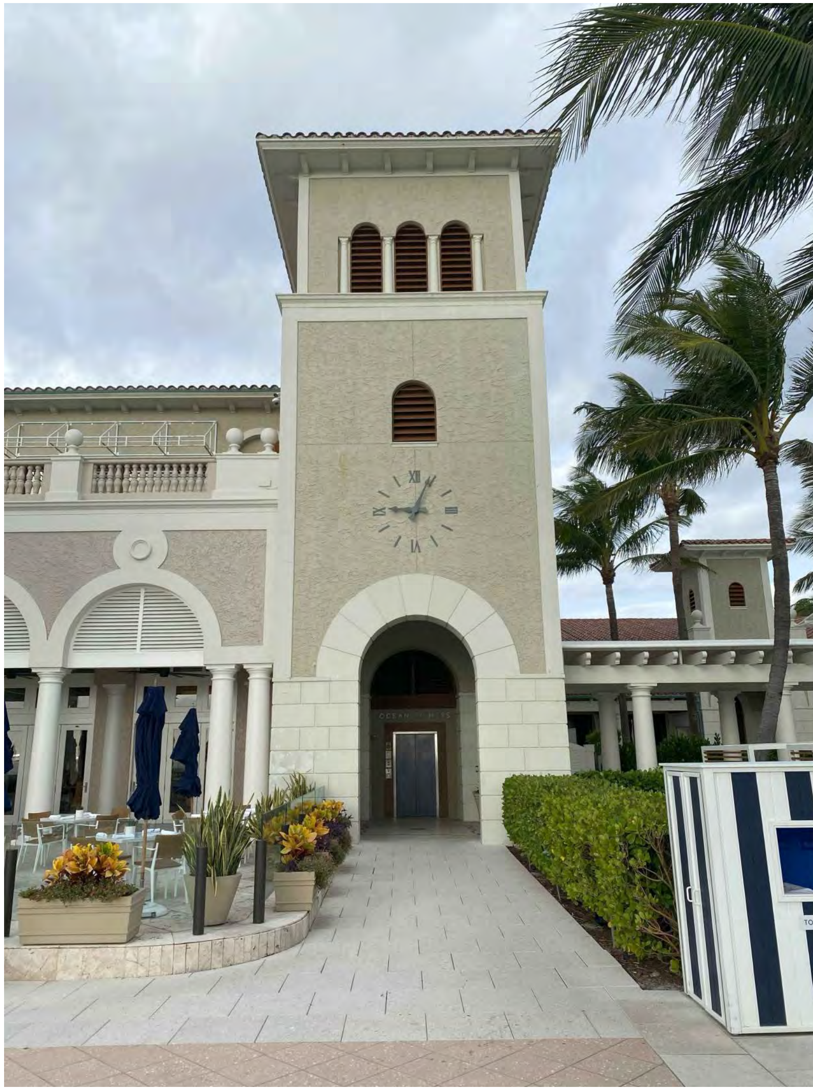
3- EXISTING OUTDOOR ENTRY TOWER EAST ELEVATION
