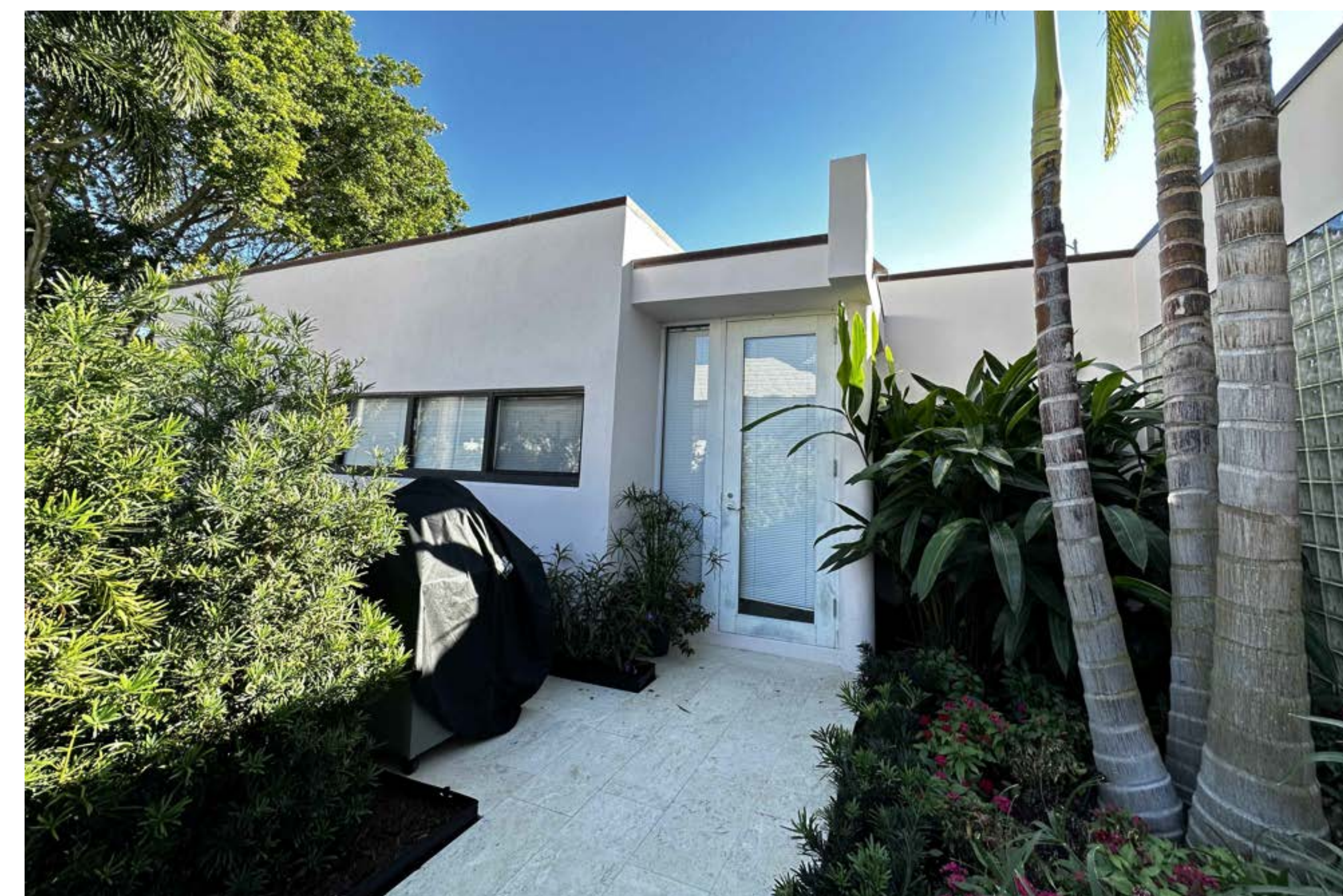
288 Sandpiper Drive West Elevation Subject Property
