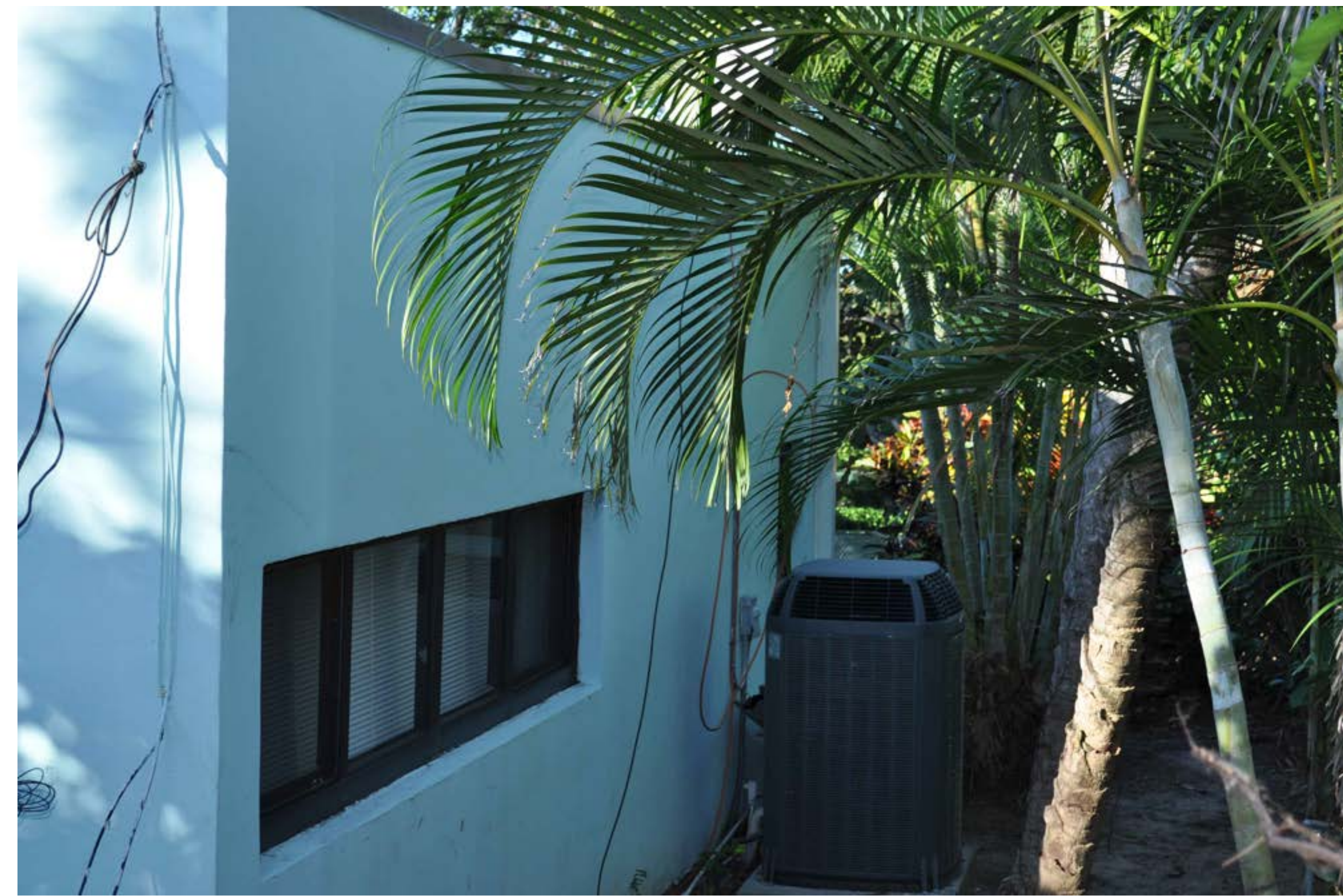
288 Sandpiper Drive East Elevation Subject Property
