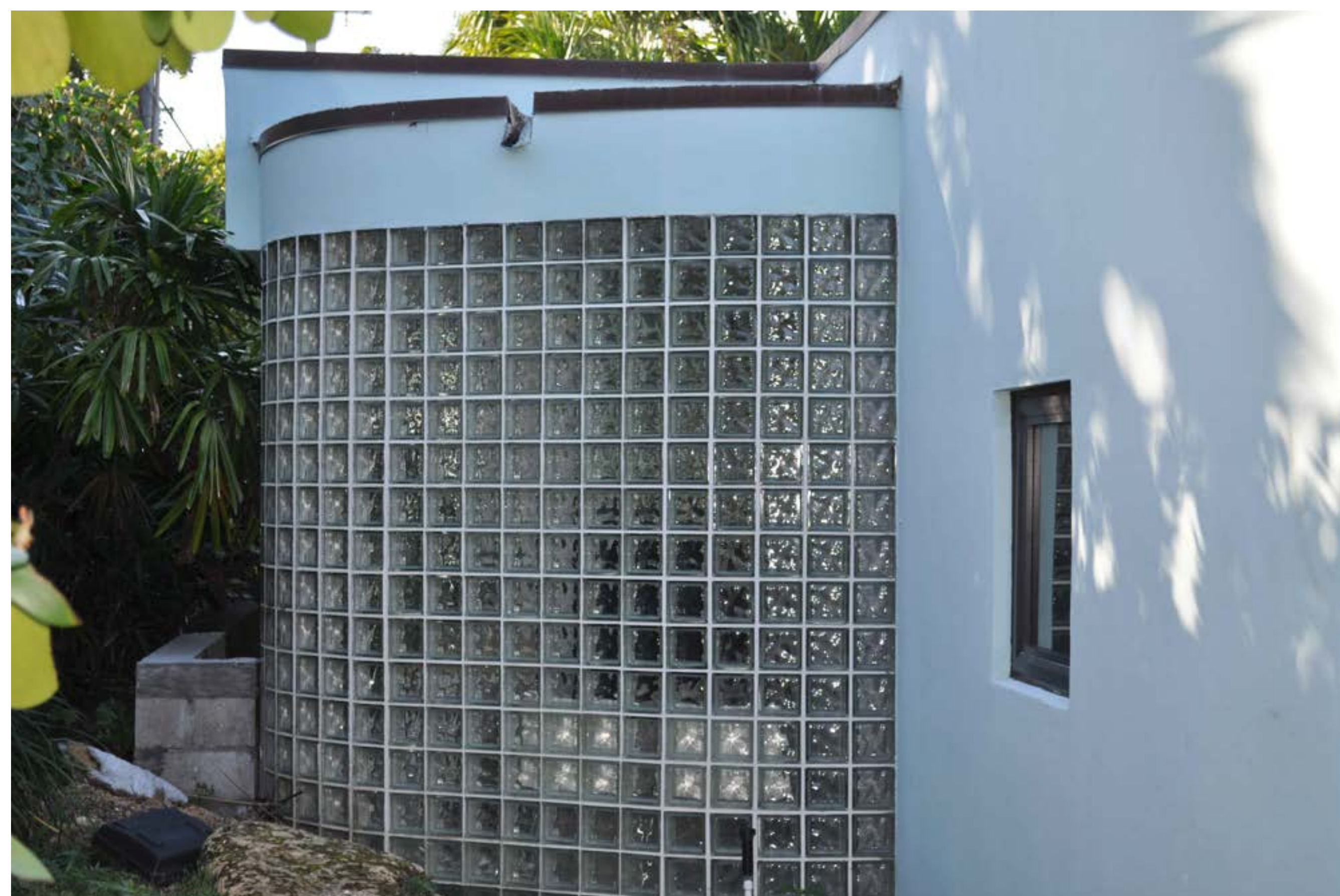
288 Sandpiper Drive East Elevation Subject Property
