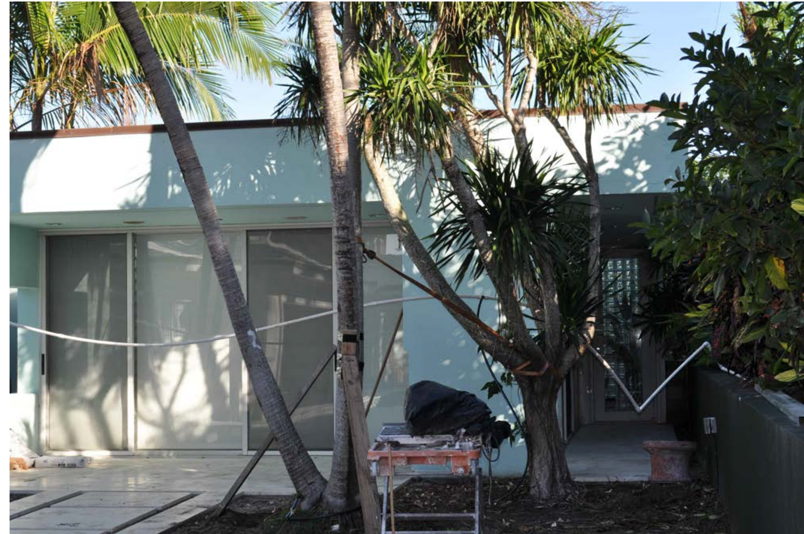
288 Sandpiper Drive West Elevation Subject Property
