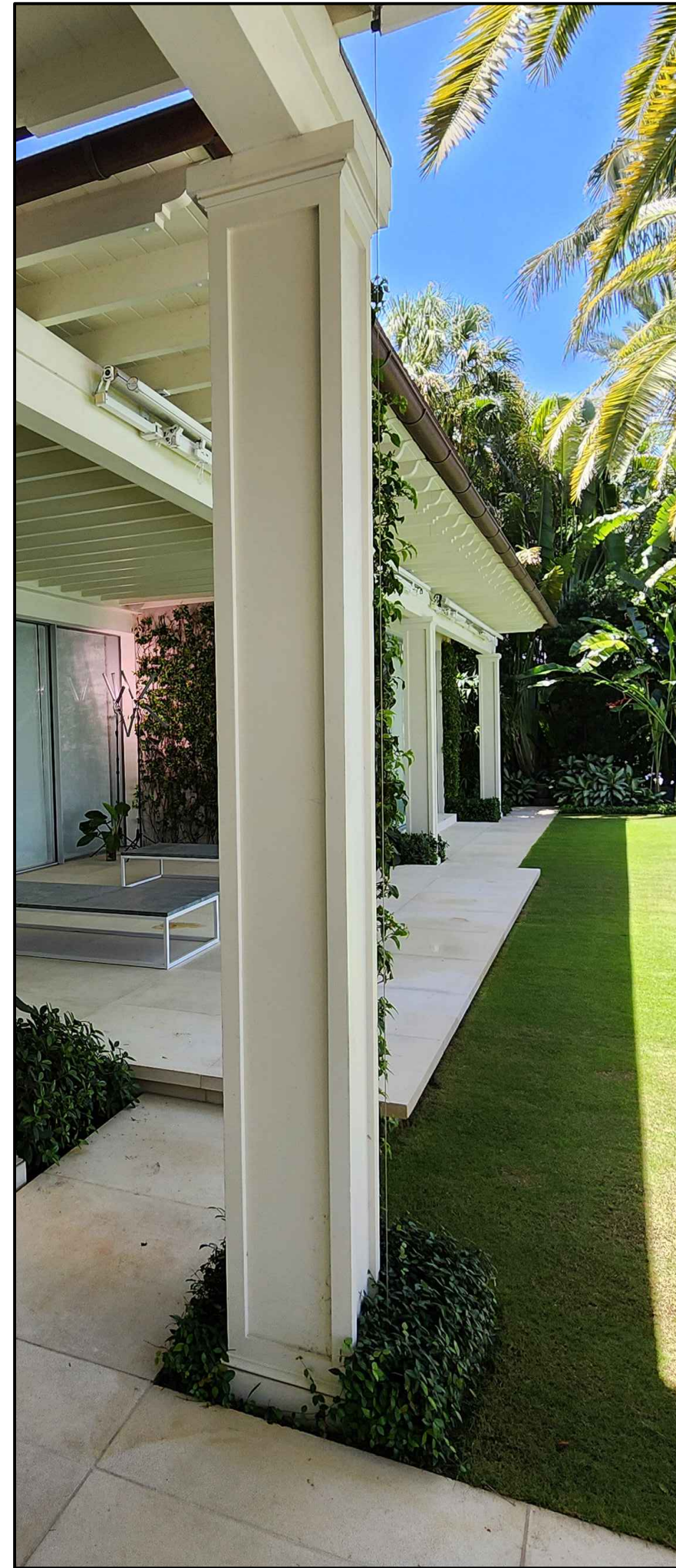
TO MATCH EXISTING Boxed-Out Columns at Loggia
