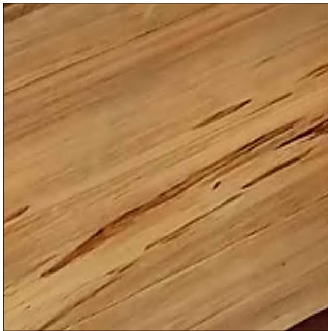
5 LIMED CYPRESS PORCH CEILINGS AT EAST COVERED PORCHES (BOTH LEVELS)
