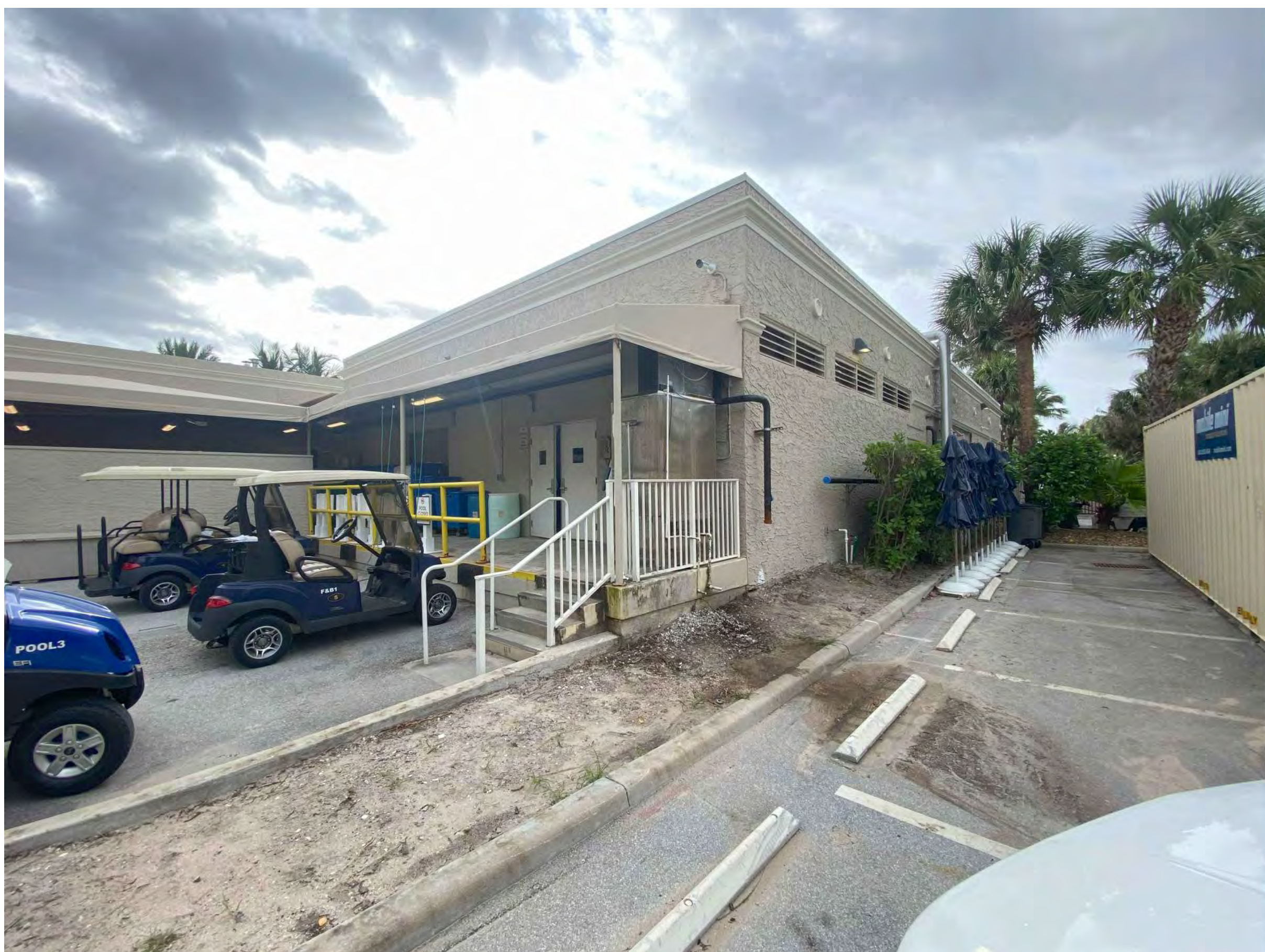
5- EXISTING LOADING ZONE LOOKING SOUTHEAST
