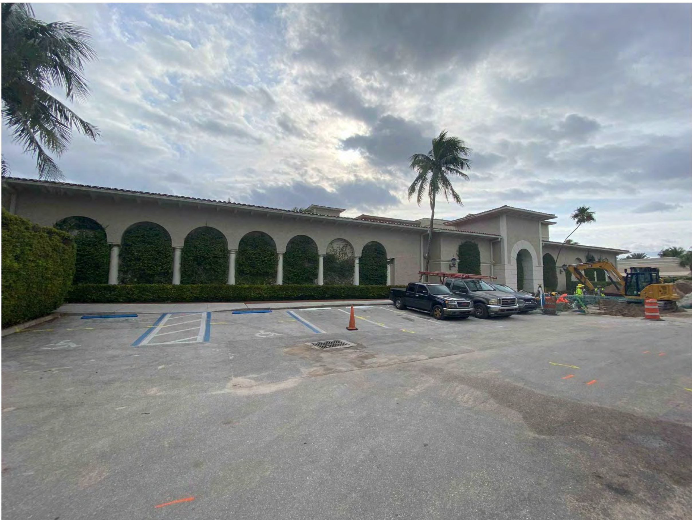
1- EXISTING PARKING LOT LOOKING SOUTHEAST
