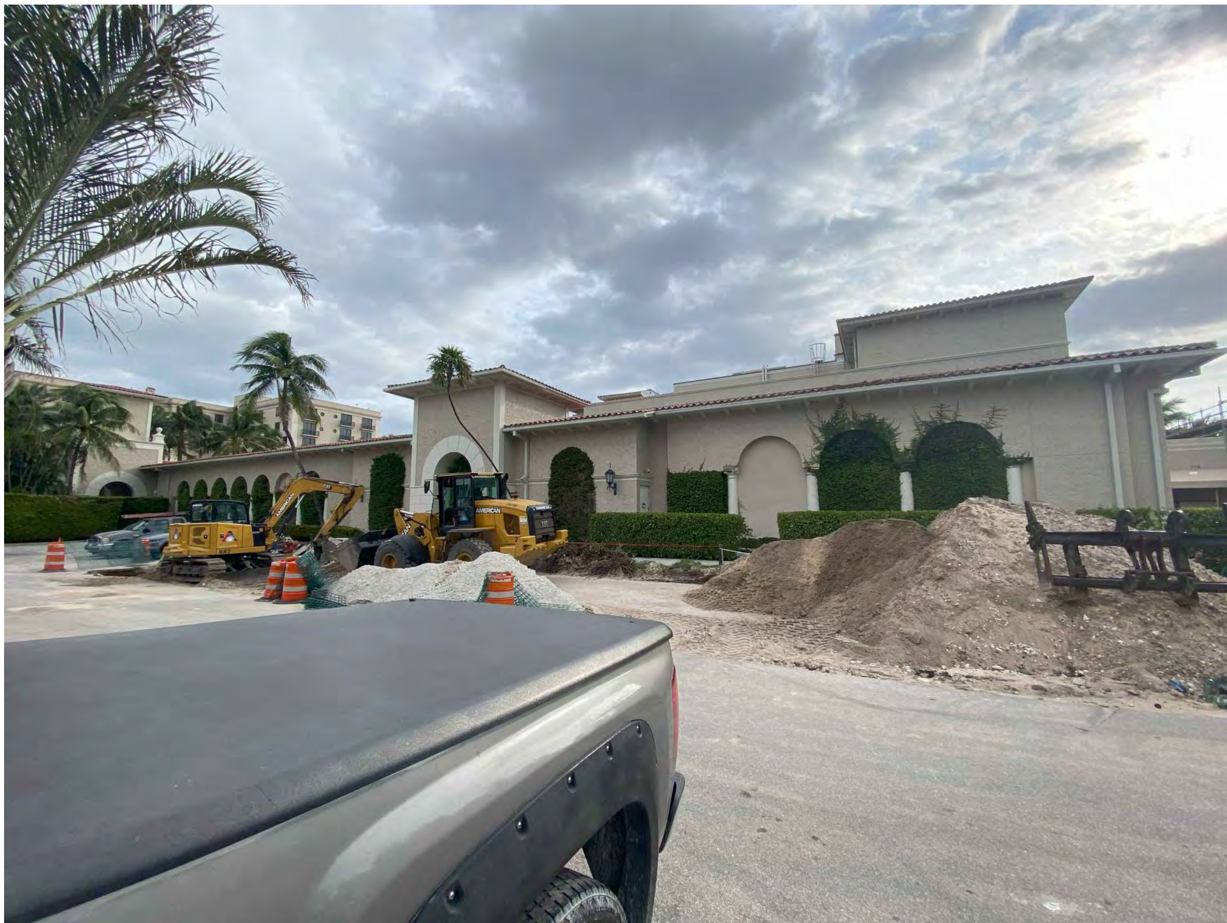
2- EXISTING PARKING LOT LOOKING NORTHEAST
