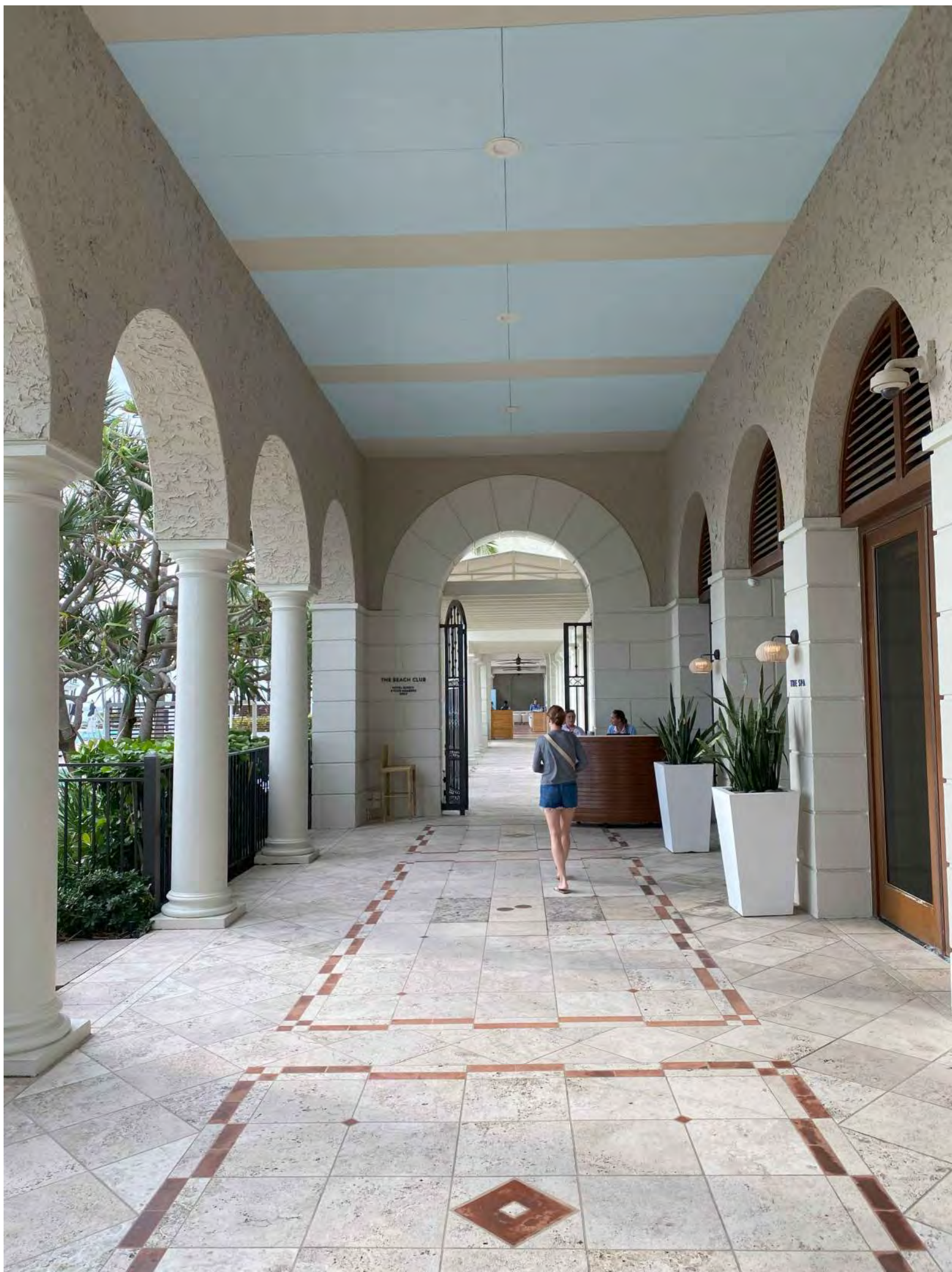
2- EXISTING SPA ARCADE ALOOKING SOUTH
