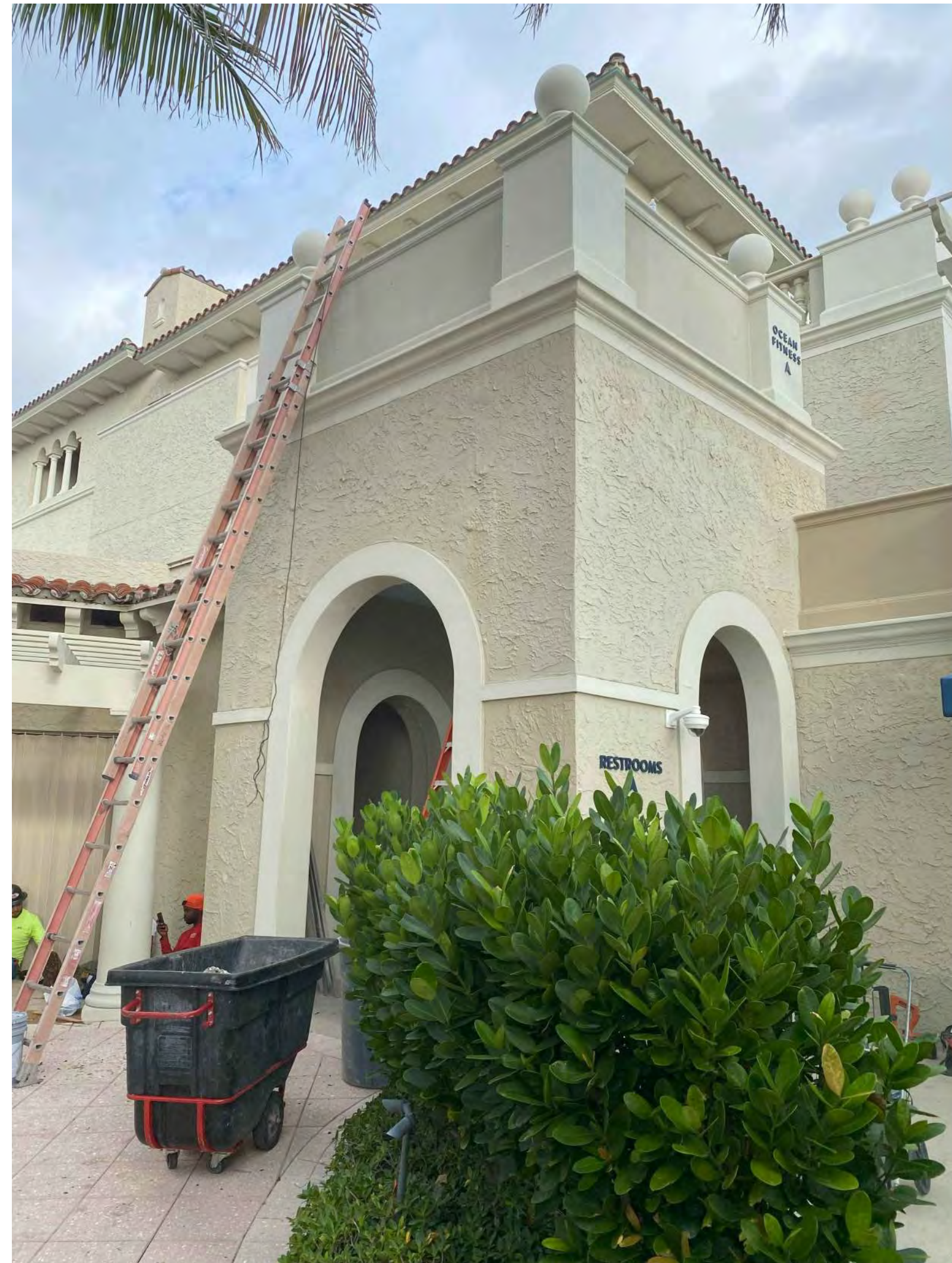
1- EXISTING RESTROOM ENTRY LOOKING NORTHWEST
