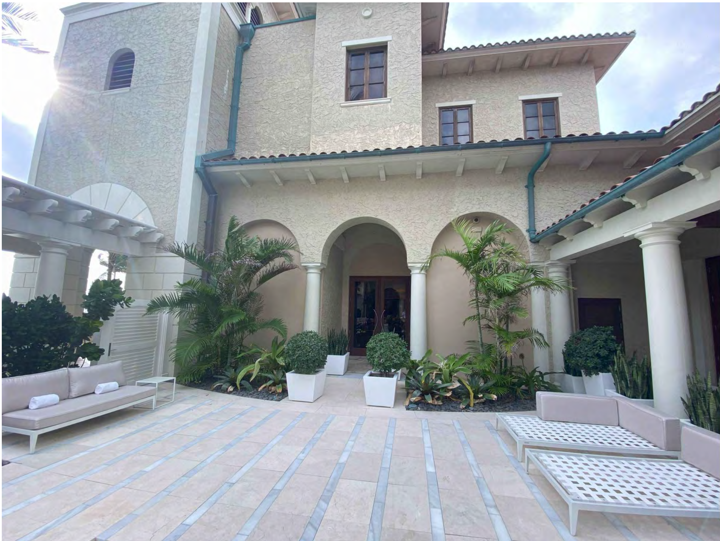
2- EXISTING SPA COURTYARD LOOKING SOUTH
