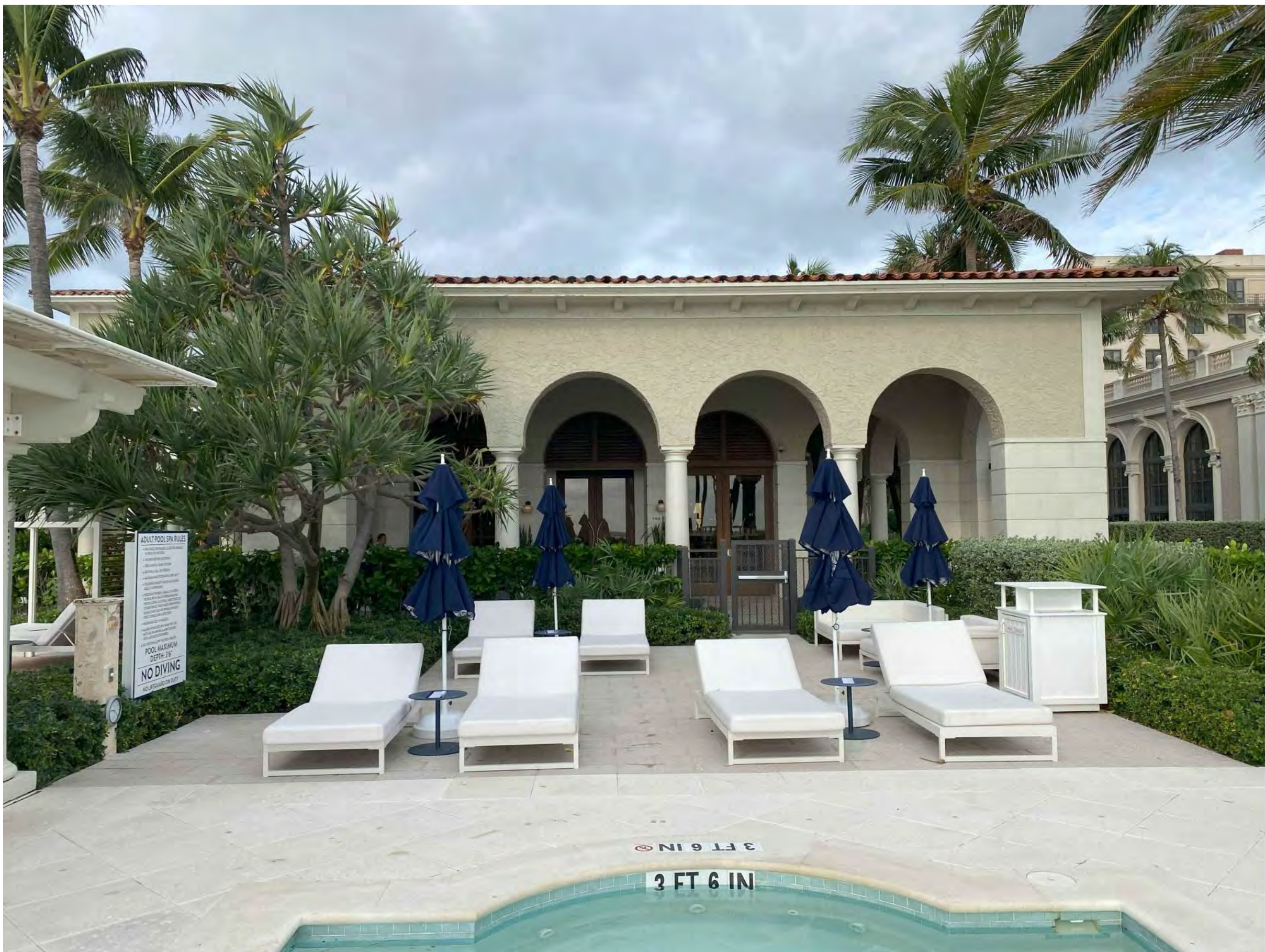
5- EXISTING WHIRPOOL ZONE LOOKING WEST
