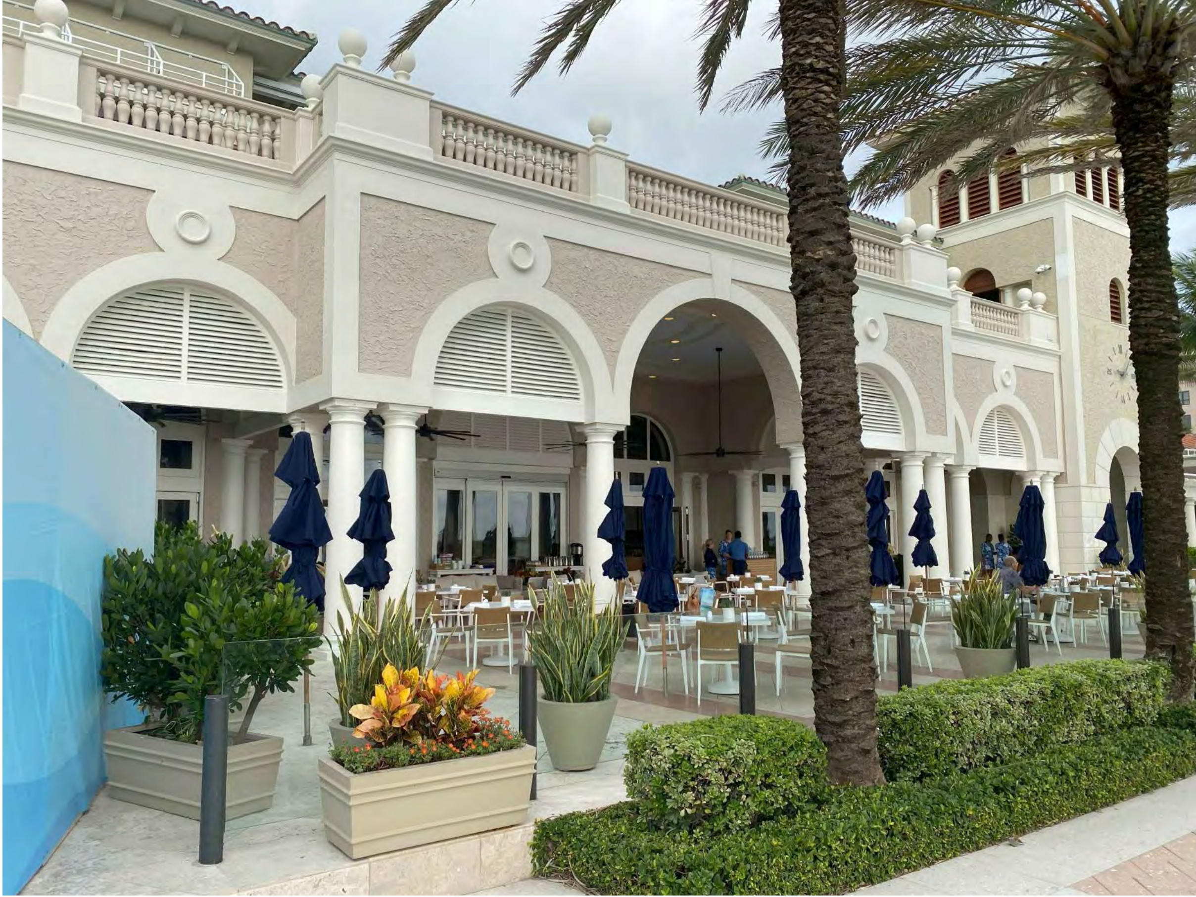
5- EXISTING OUTDOOR DINING LOOKING NORTHWEST
