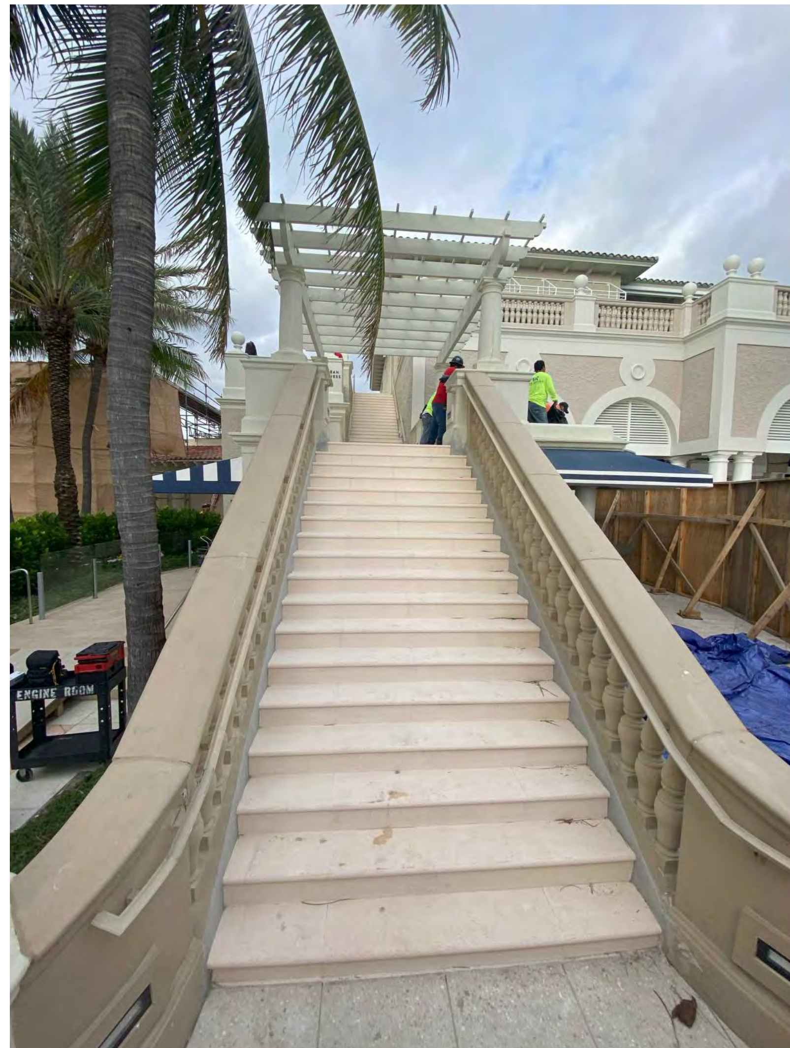
4- EXISTING STAIRWAY TO OCEAN FITNESS
