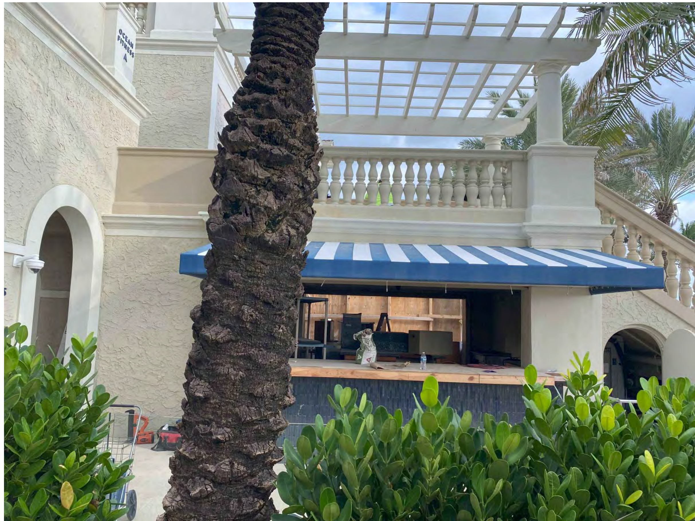
2- EXISTING OUTDOOR BAR LOOKING NORTH
