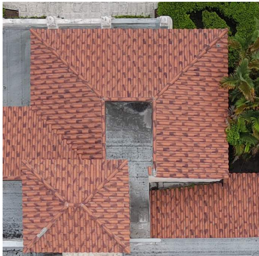
CLAY BARREL TILE, TRADITIONALLY DETAILED
