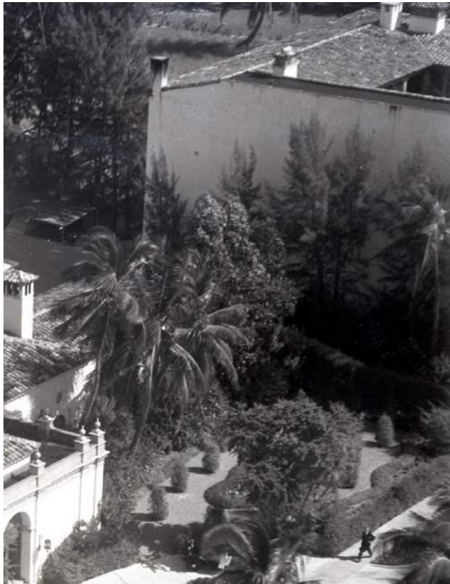
HISTORIC AND EXISTING PHOTO - WEST ELEVATION
