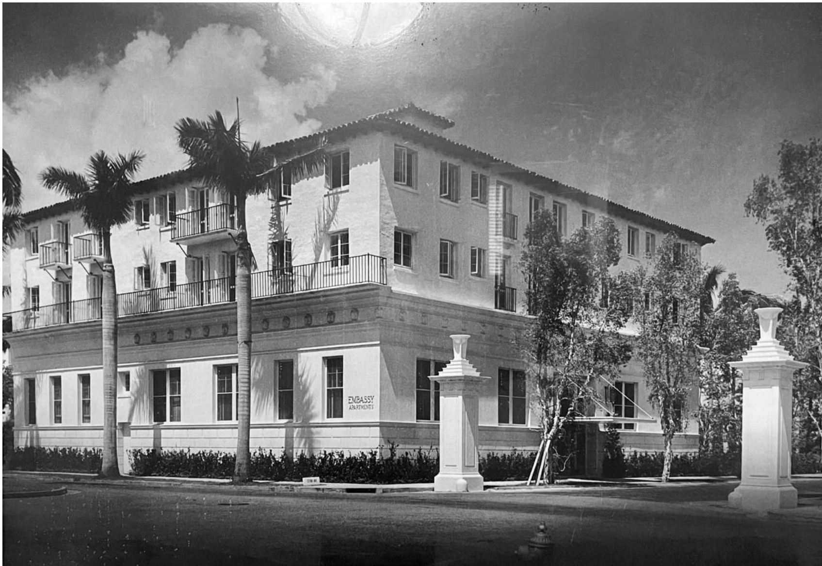
5 PHOTOGRAPH OF EXTERIOR, SOUTHEAST CORNER, CIRCA 1947
