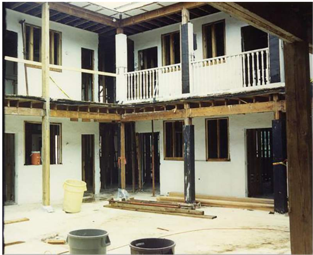
3 PHOTO - COURTYARD PRIOR TO DEMOLITION, 1992
