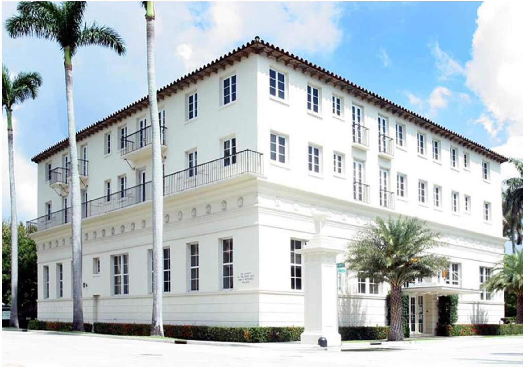
4 PHOTOGRAPH OF EXTERIOR, SOUTHEAST CORNER, CIRCA 1947
