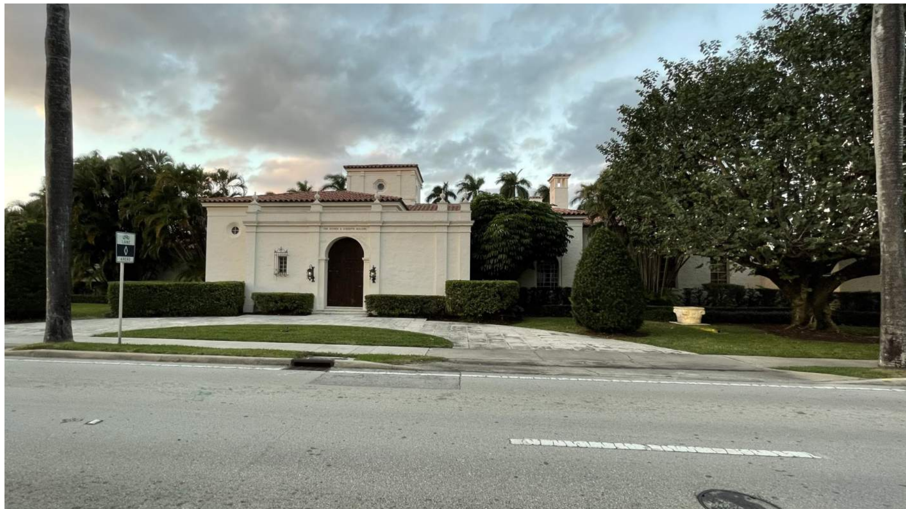
EXISTING PHOTOS - SOUTH ELEVATION
