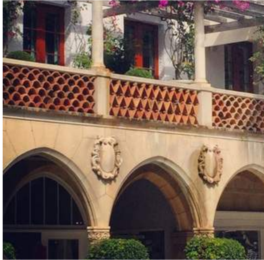
FISH SCALE BARREL TILE (EAST ROOF VENTILATOR ENCLOSURE)
