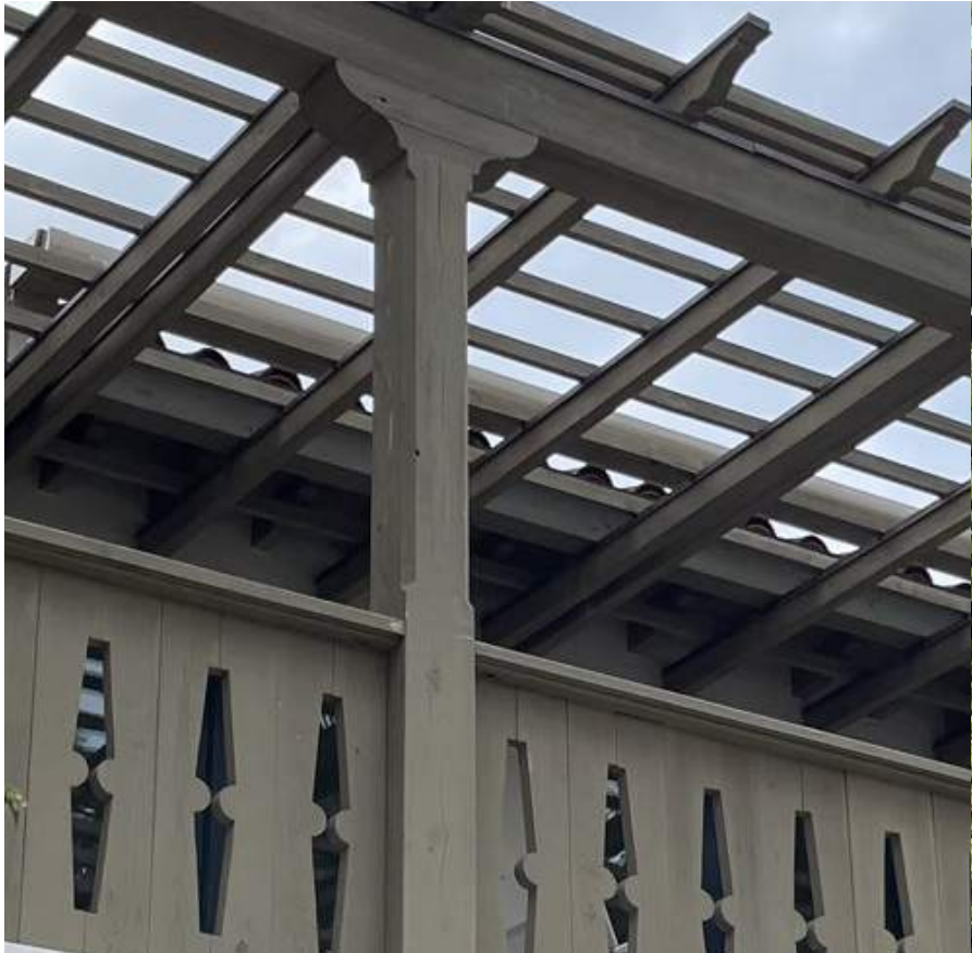
SOUTH LOGGIA - OLD-GROWTH CLEAR CYPRESS, LIME WASH
