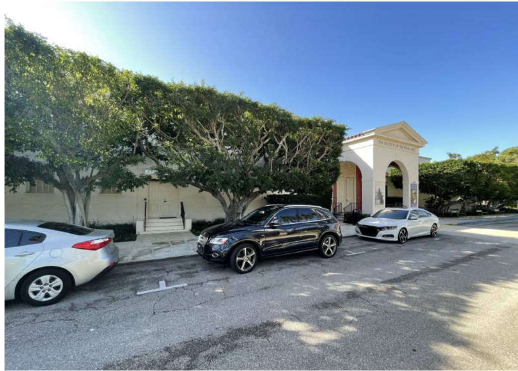
EXISTING PHOTOS - NORTH ELEVATION
