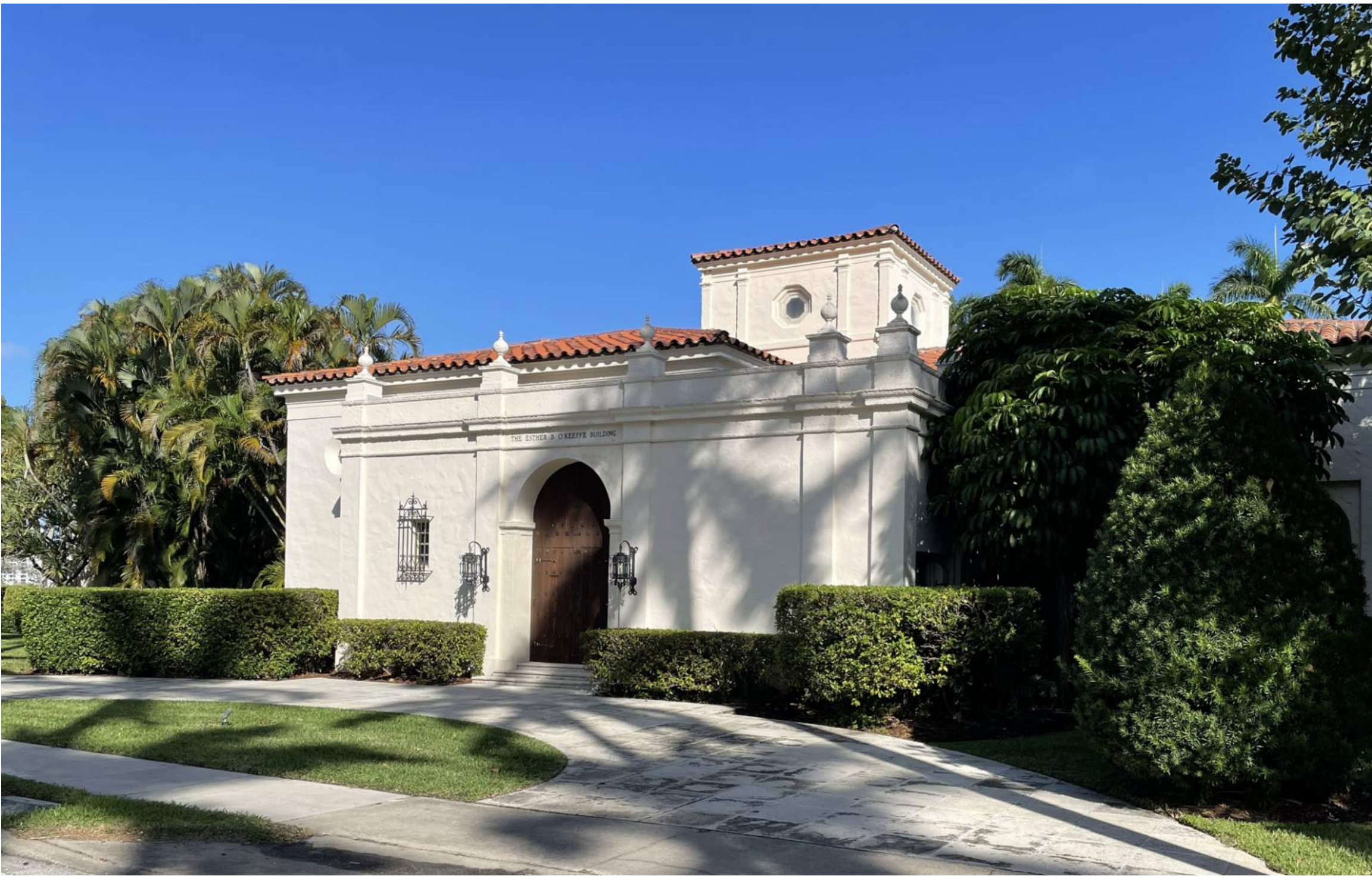
4 EXISTING PHOTOGRAPH, LOOKING NORTHWEST FROM ENTRANCE B-4.6.2 NTS
