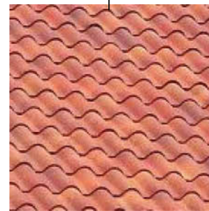
CLAY TILE ROOF
