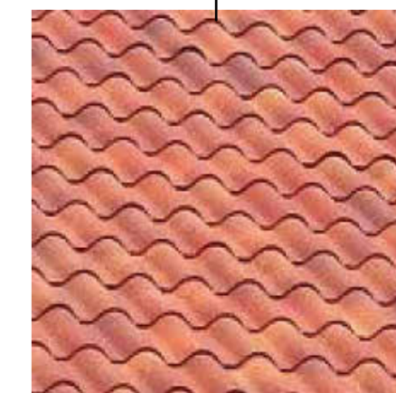
CLAY TILE ROOF
