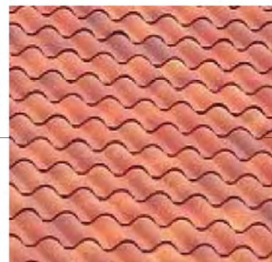
CLAY TILE ROOF
