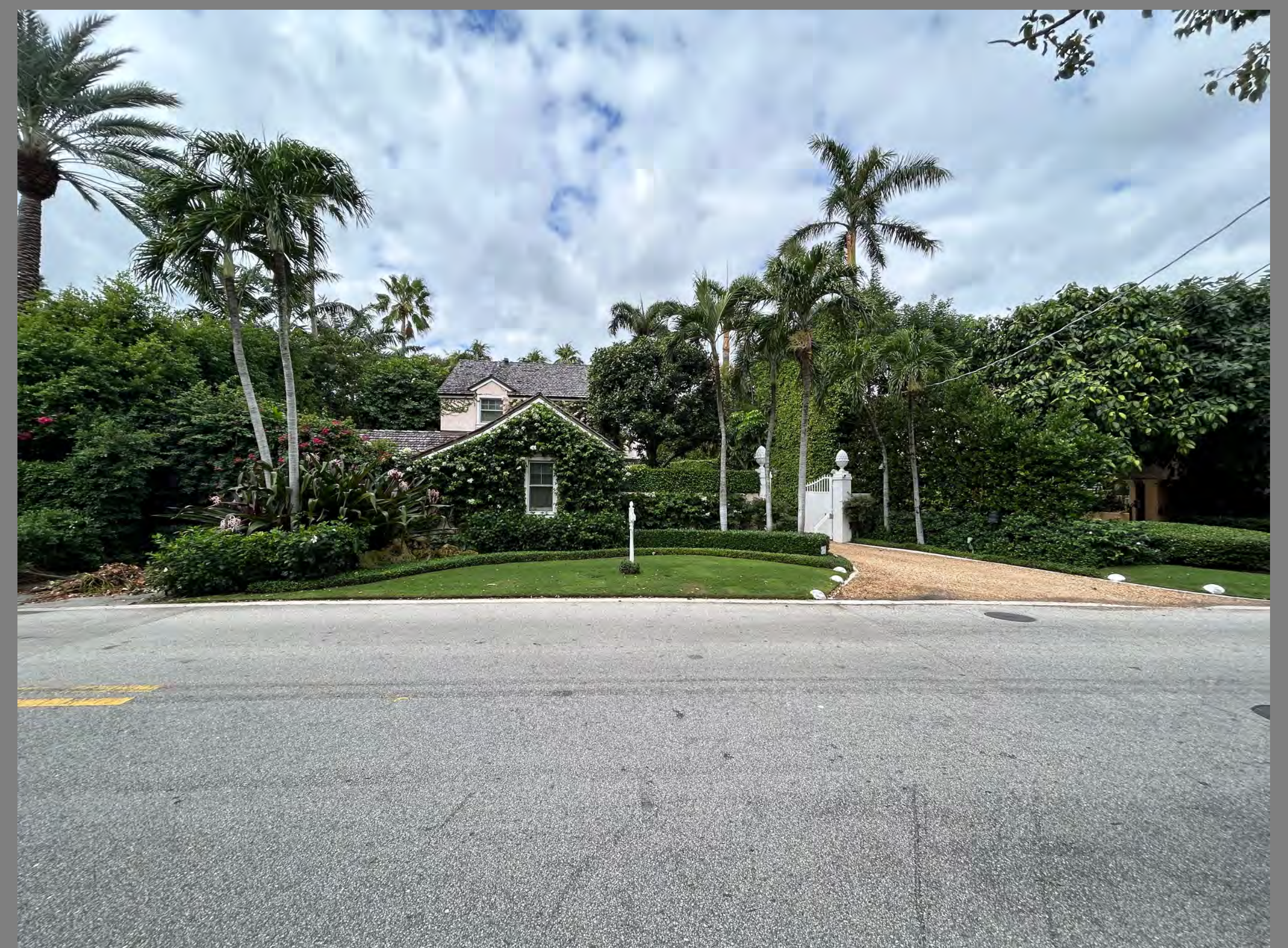
2 STORY GUEST HOUSE AT SUBJECT PROPERTY
