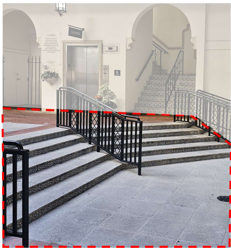
Replacing pavers on steps with new hand-painted decorative tile at risers. Existing railings to remain until future phase of project.
