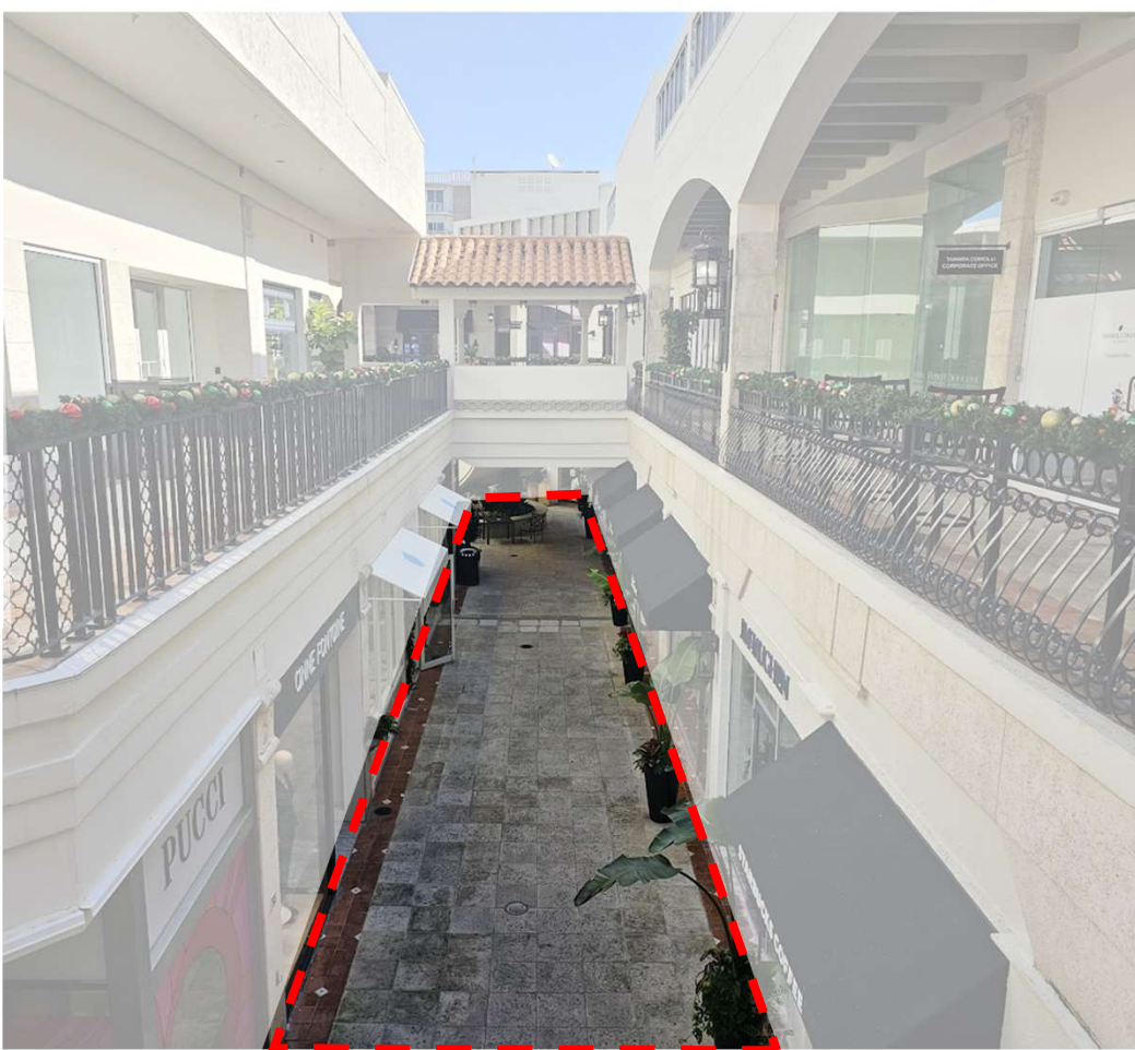
Replacing existing pavers with new pavers as part of waterproofing project, replacement of new drains while keeping existing drainage pipes.
