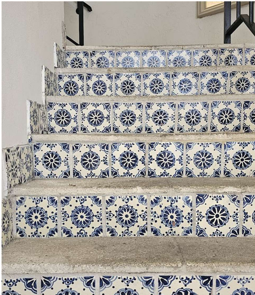
Tile at Original Egress Stairs Likely Original
