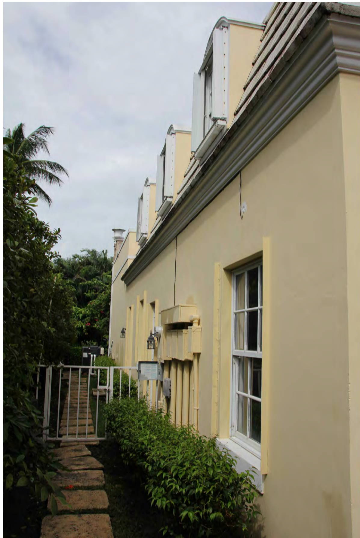
SOUTH SIDE OF PROPERTY
