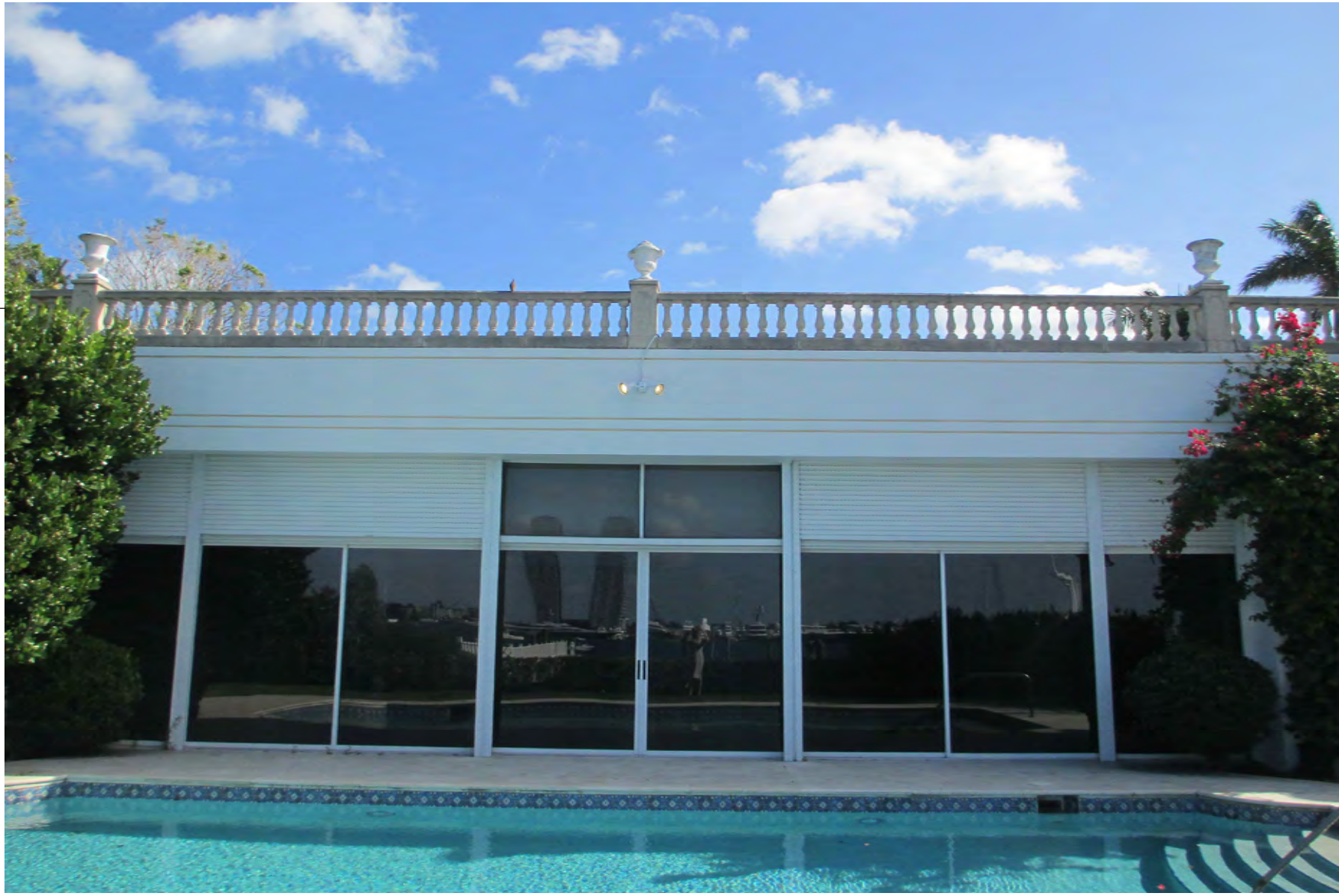
WEST SIDE OF PROPERTY
