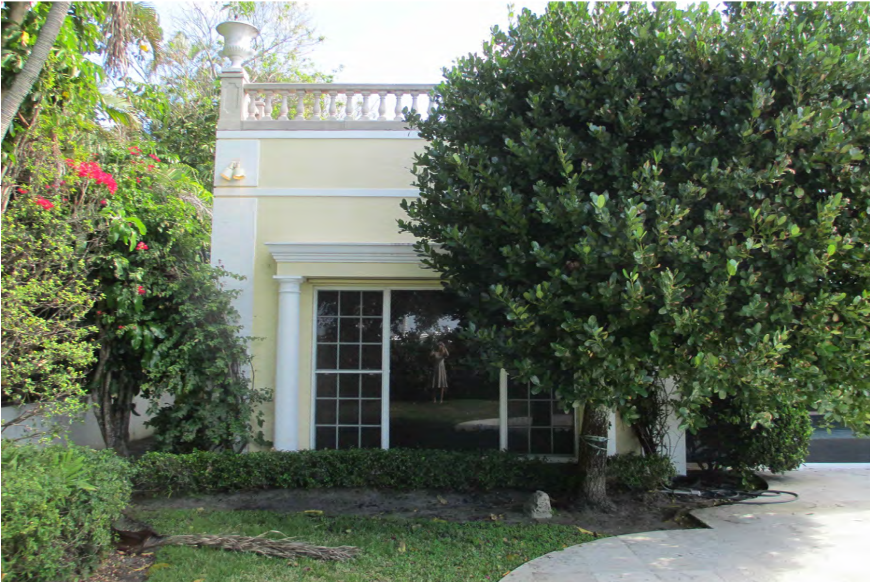
WEST SIDE OF PROPERTY
