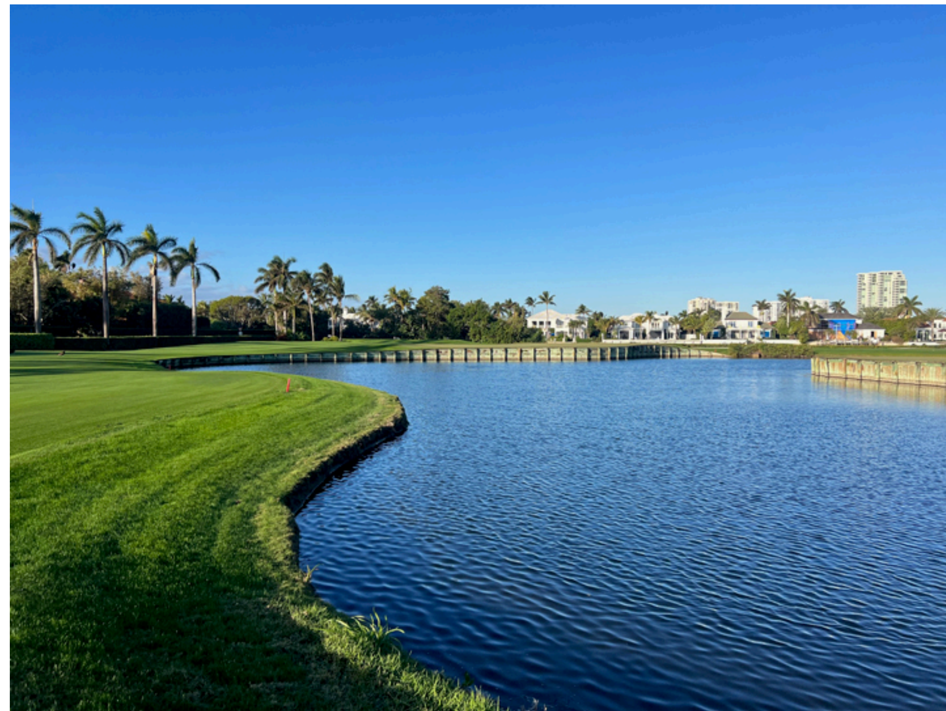
#2 green from the fairway. We will remove most of the bulkheads on the course, like the one pictured here. The shoreline at the green will resemble the foreground and will be grassed with Seashore Paspalum at a 4-1 slope from the fairway to the waters edge. Paspalum is the best grass for this area because it is salt tolerant and most of the lakes contain brackish water. This area will be maintained at rough height to properly follow the protocol Florida's BMP's for Water Quality.
