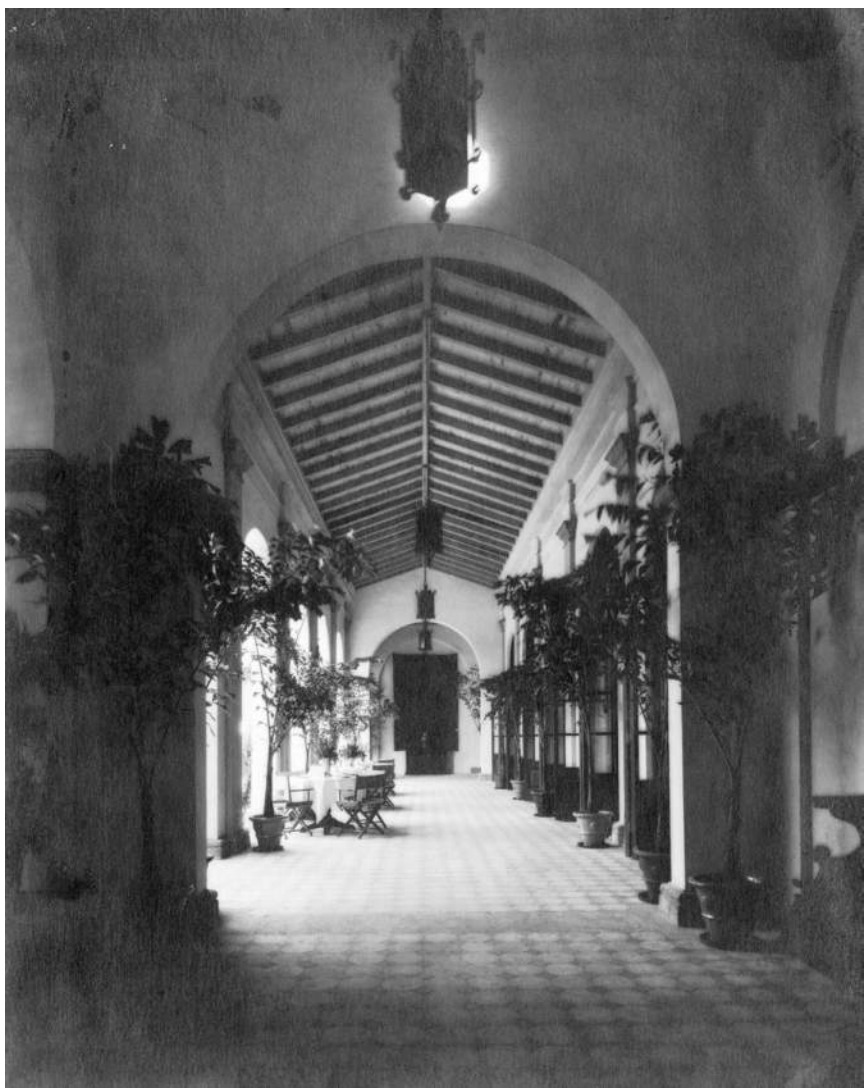
3 PHOTO - CENTRAL LOGGIA, LOOKING NORTH, CIRCA 1930 B-1.0.0 NTS - COURTESY HISTORICAL SOCIETY OF PALM BEACH COUNTY
