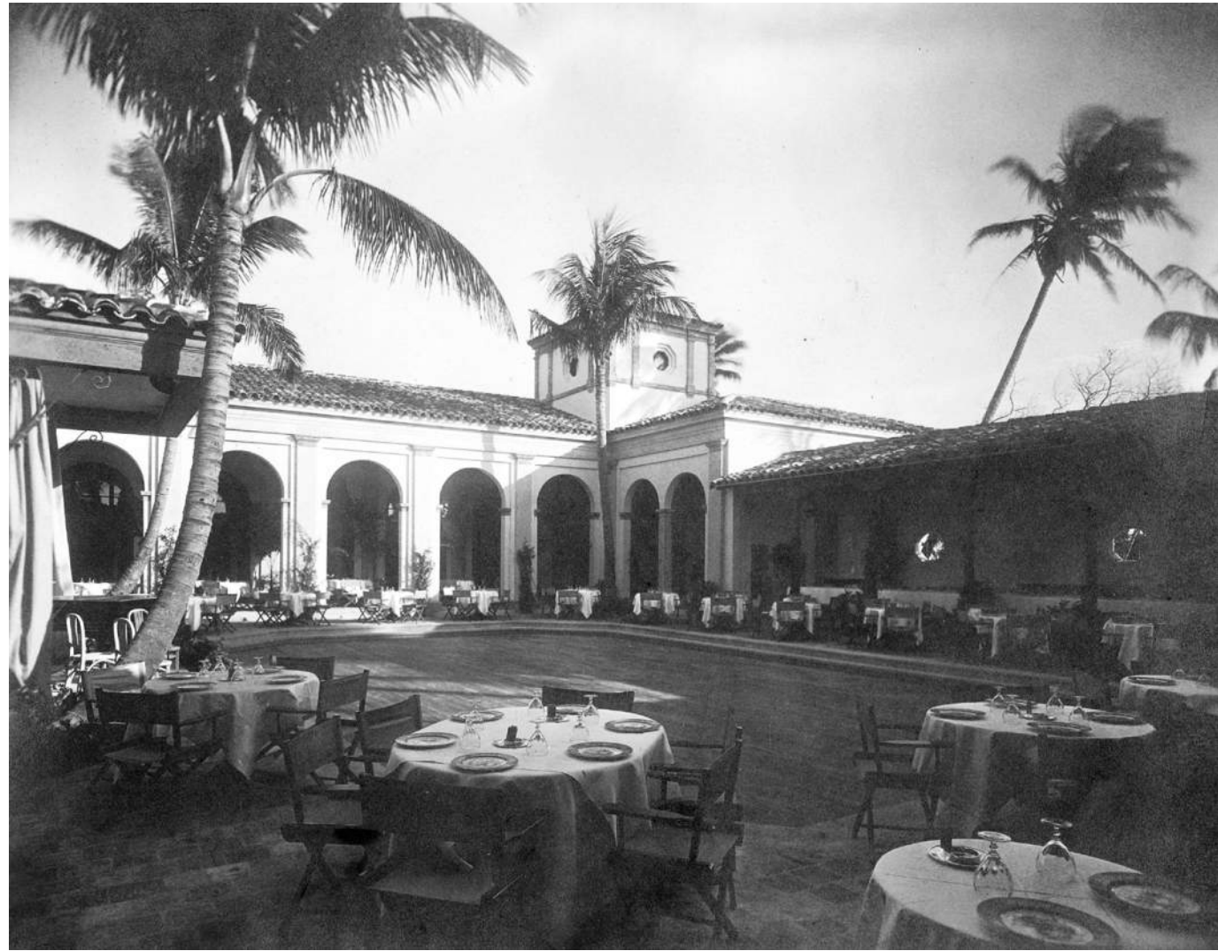
5 PHOTO - LOGGIA AND SOUTH CLOISTER FROM PATIO, CIRCA 1930 B-1.0.0 NTS - COURTESY HISTORICAL SOCIETY OF PALM BEACH COUNTY
