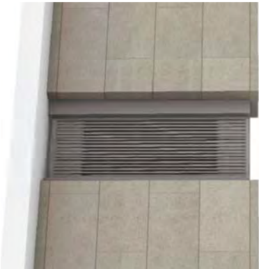
VIEW: SERVICE GATE AT BATH GARDEN WEST WALL
