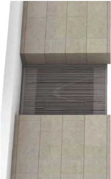
VIEW: SLIDING GATE AT BATH GARDEN EAST WALL
