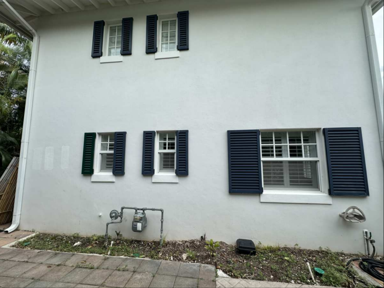
G) west property line looking east
