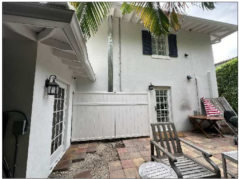
E) north property line looking south
