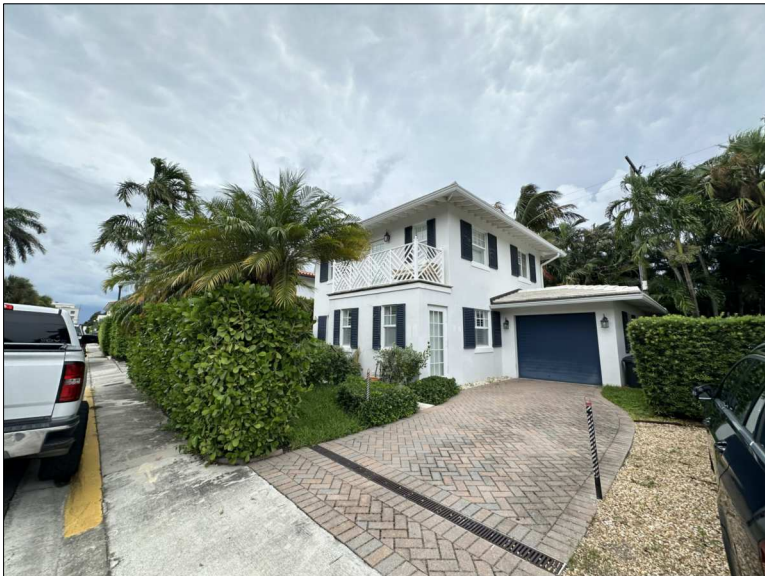
B) southeast corner looking northwest
