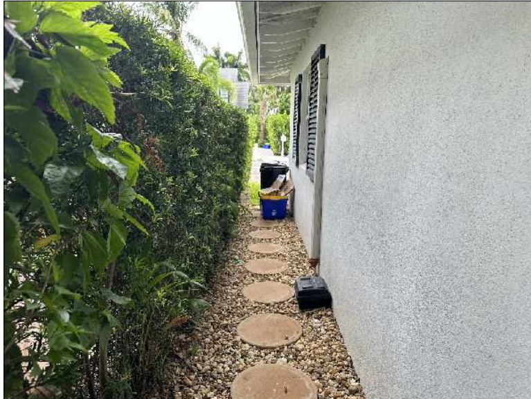
C) northeast corner looking south
