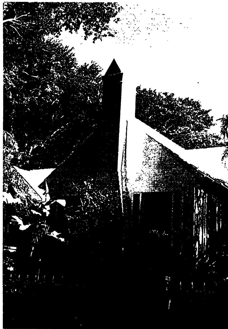
Full length chimney with windcap
