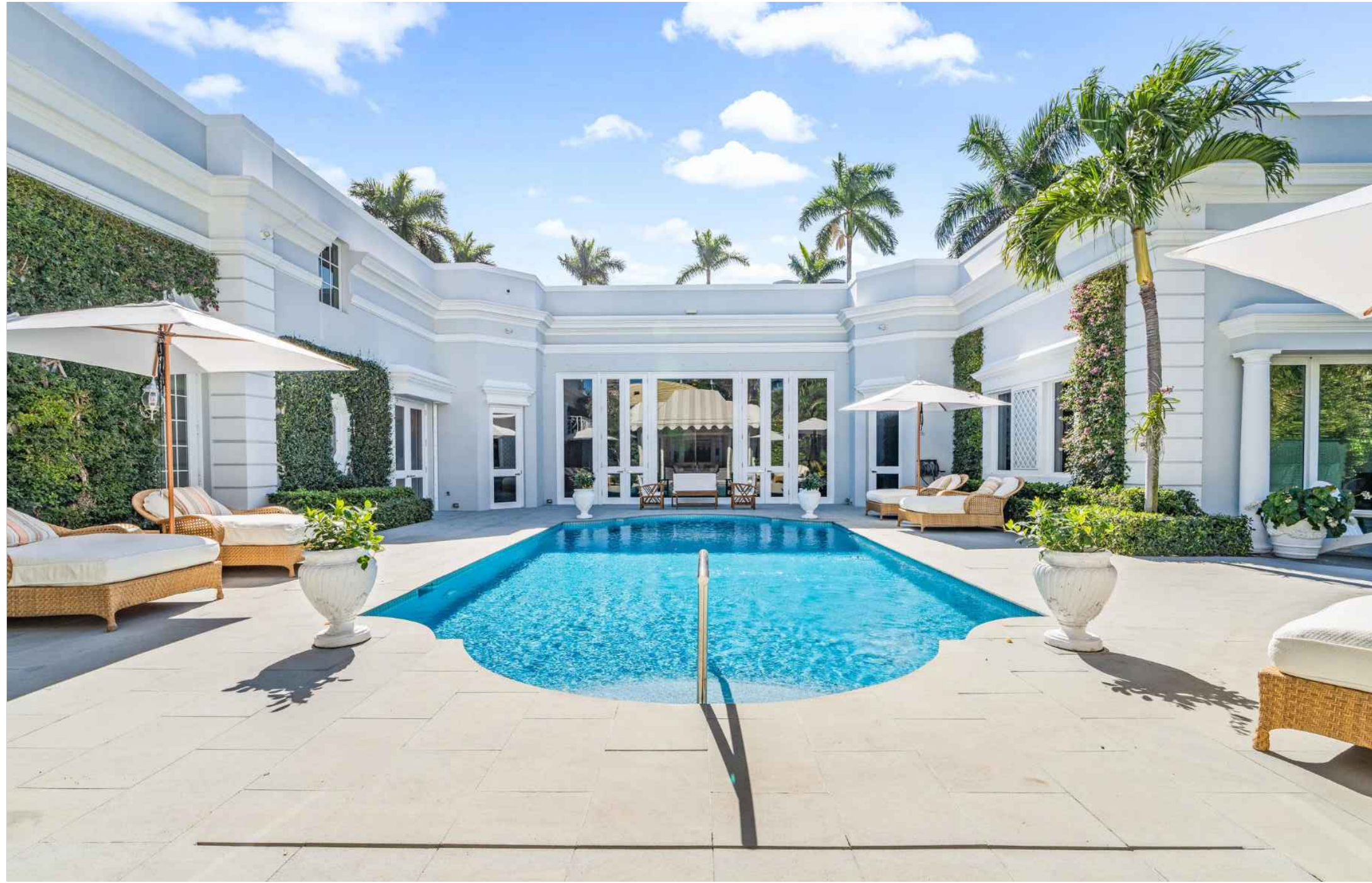
01-COURTYARD LOOKING SOUTH
