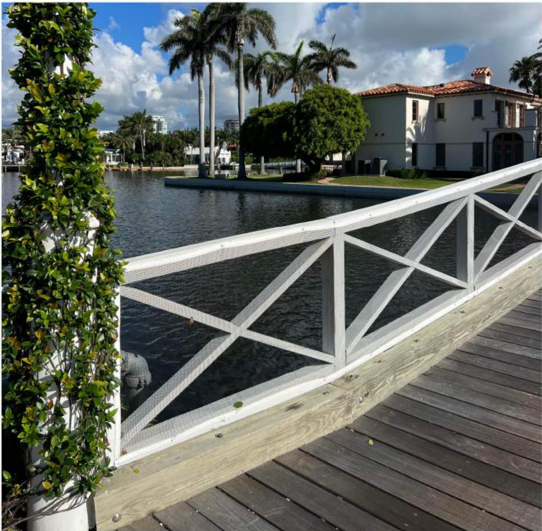
NORTH ENTRY BRIDGE
