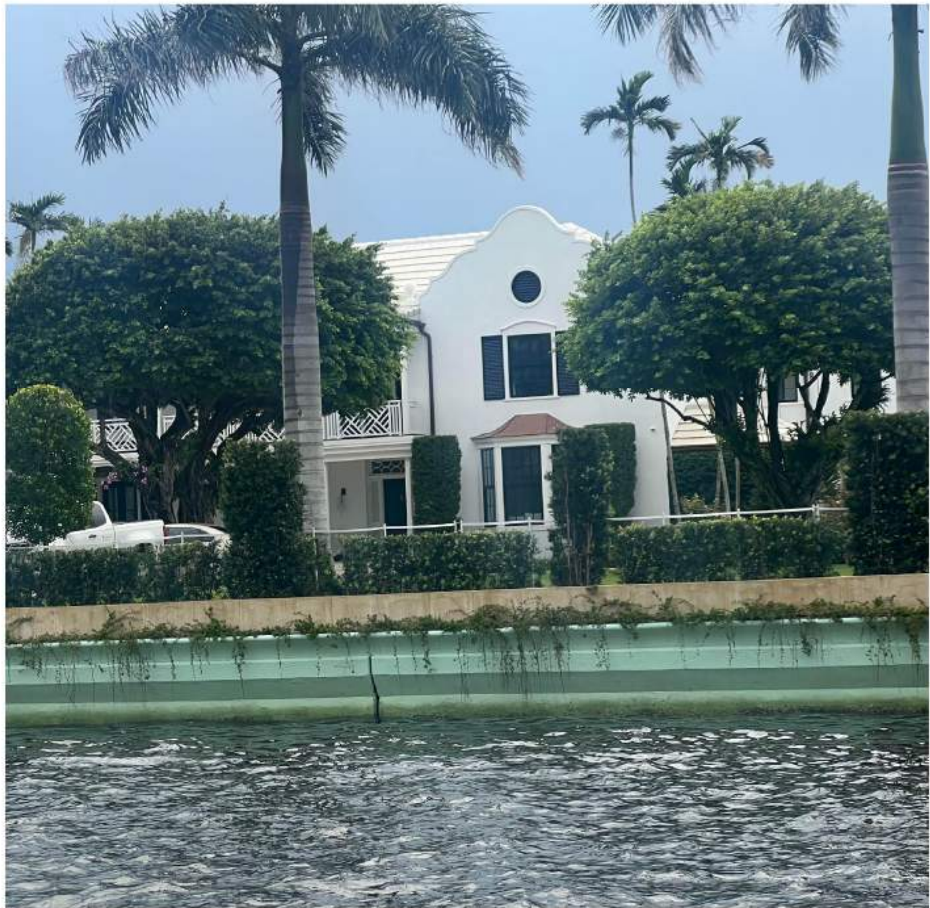
SEA WALL AT FRONT YARD
