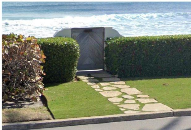
The current gate is made of diagonal wood pieces with flared stucco end caps leading to the sea wall. This gate matches the materials of an entry gate on the south side of the property.
