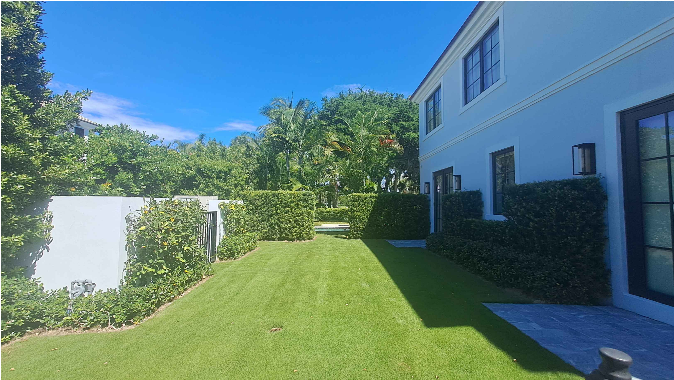
Front view / South (Existing)
