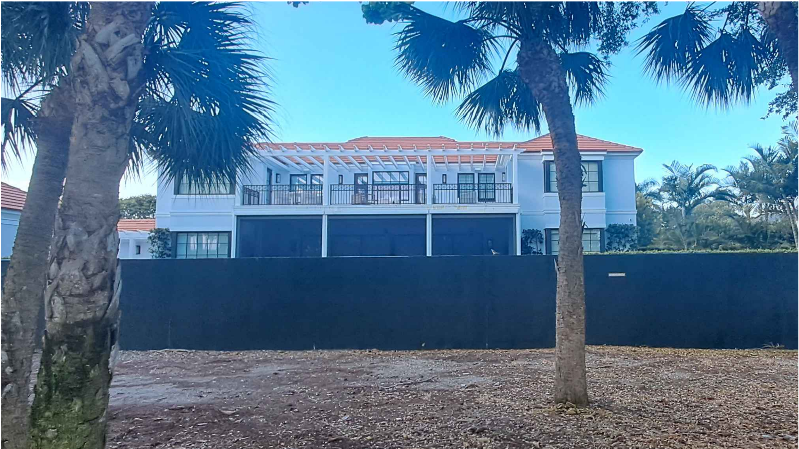
North View / Golf Course View
