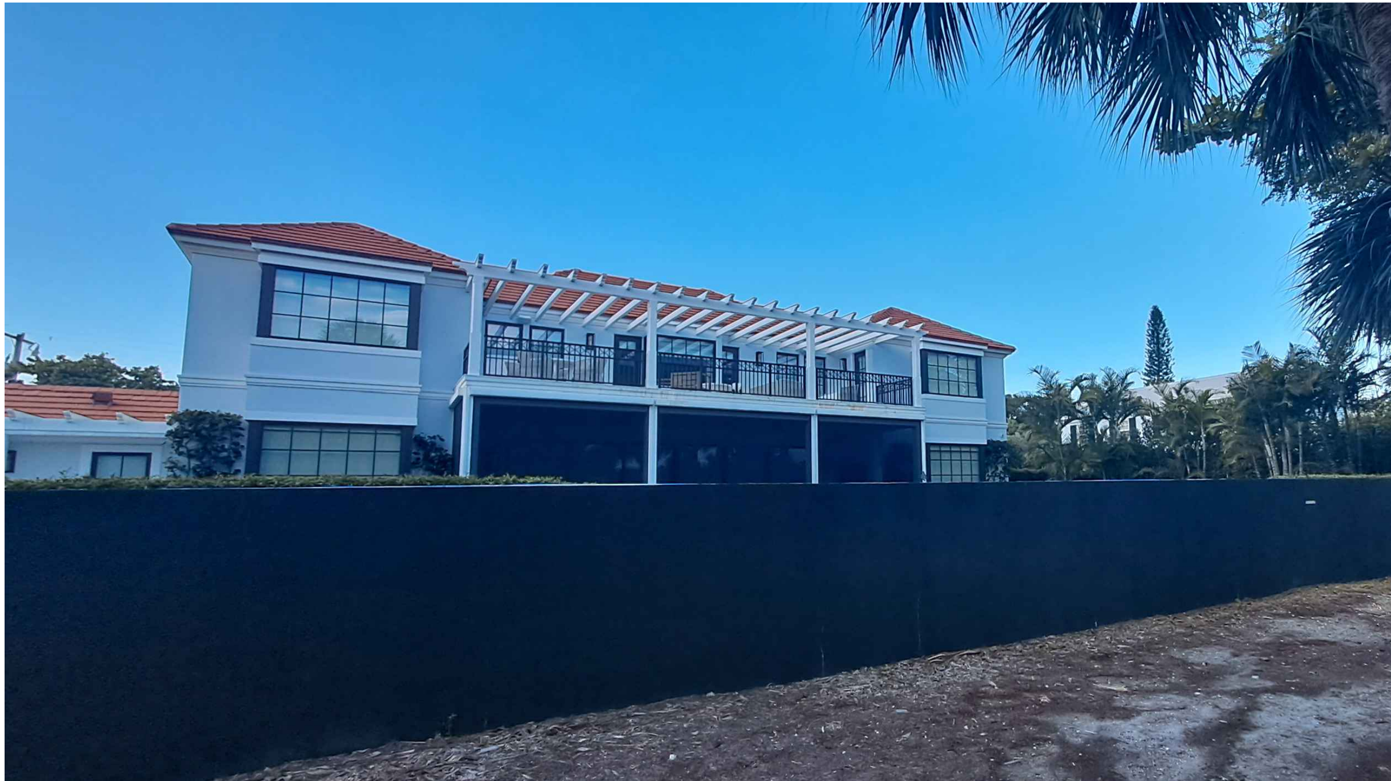
North View / Golf Course View
