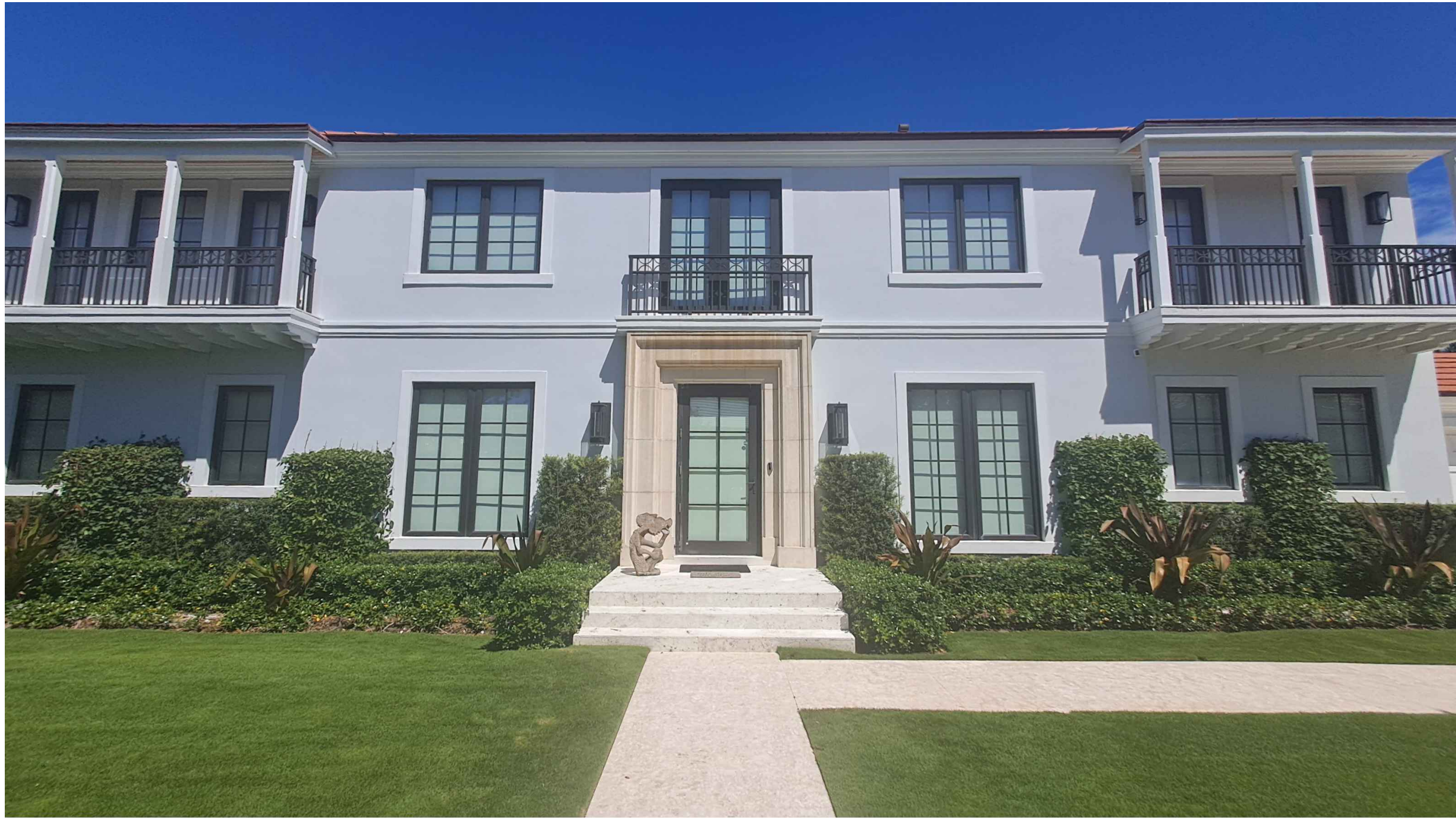
Front view / South (Existing)
